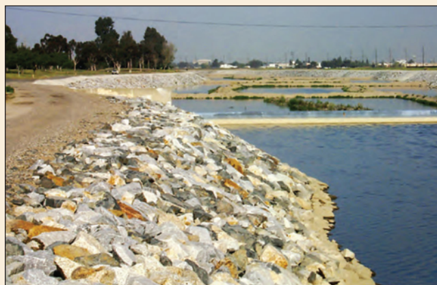
Recharge basins infiltrate Santa Ana River water into the aquifer
