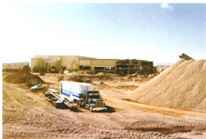
Figure 8. On-site recycling of demolition debris for use as aggregate at the former Cinderella City shopping mall in Denver, Colo.
