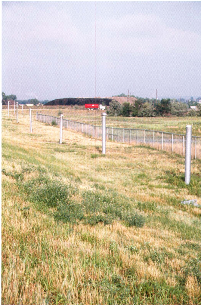
Figure 22. An older sanitary landfill in an exhausted sand and gravel pit near Interstate 76 and Pecos Street requires vents to allow methane gas to escape. Methane is generated from decomposing organic matter in landfill and its presence precludes other uses of land in near future.
