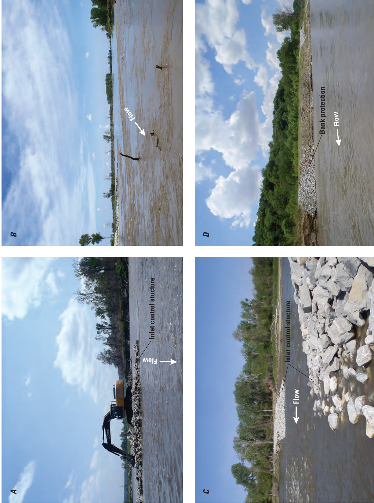
Figure 2. Control structures at Missouri River chutes, 2011–13. A , Construction of a new inlet control structure at Derooin chute, 2013. B , Turbulent water around the inlet control structure and snags at Lower Hamburg chute, 2014. C , New control structure within Lower Hamburg chute, 2014. D , Limited bank protection on an eroded bank at Tobacco chute, 2014.
