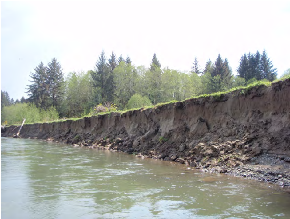
Figure 3. View looking upstream along the slumping left bank of the Quillayute River, Washington, May 4, 2010. Location of photography site shown in figure 2 , point A. Photograph taken by Christiana Barnas, U.S. Geological Survey.
