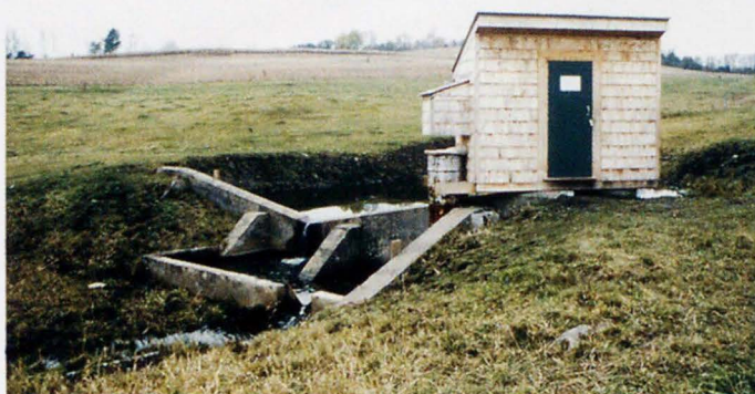
This streamflow-gaging station (W-2) records streamflow from a 59-hectare agricultural catchment. The USGS operates 4 of the original 17 Sleepers River streamgages, as well as 5 new gages on small streams within the forested headwater catchment W-9.
