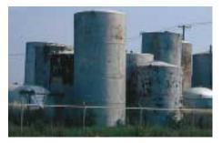
Figure 4. Abandoned tanks and pipes may contain radium in scale and sludge.
