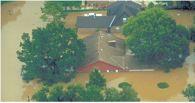
Figure 4. Land subsidence of 5 to 7 feet in a residential area in northern Houston exacerbated flooding in June 1989.
