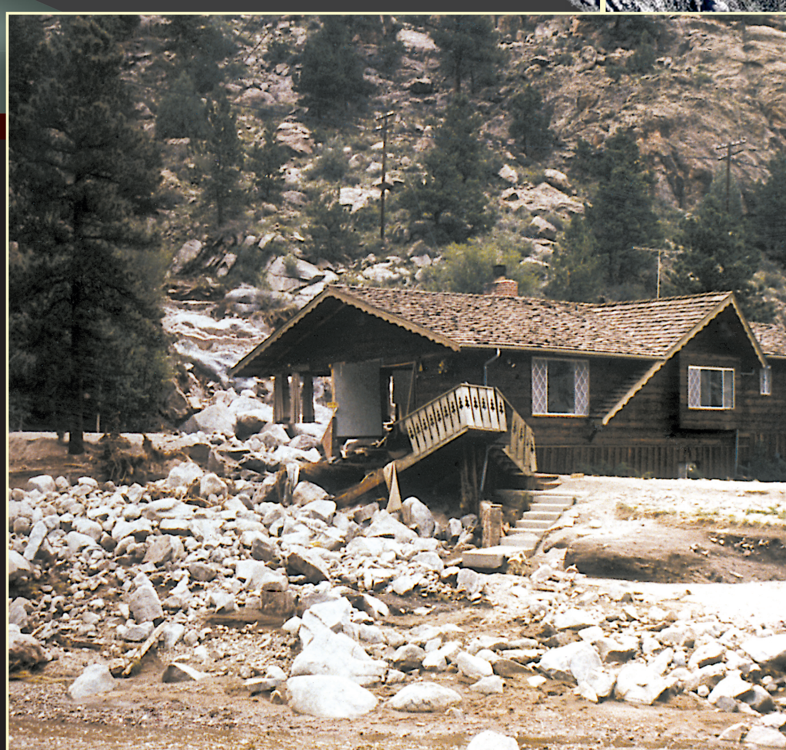
This house was built on an alluvial fan that was produced by sediment discharged from a side canyon. Floodwaters from the side canyon crushed part of the house and pushed it about 4 feet off its foundation. Mile 91.1, Big Thompson River.
