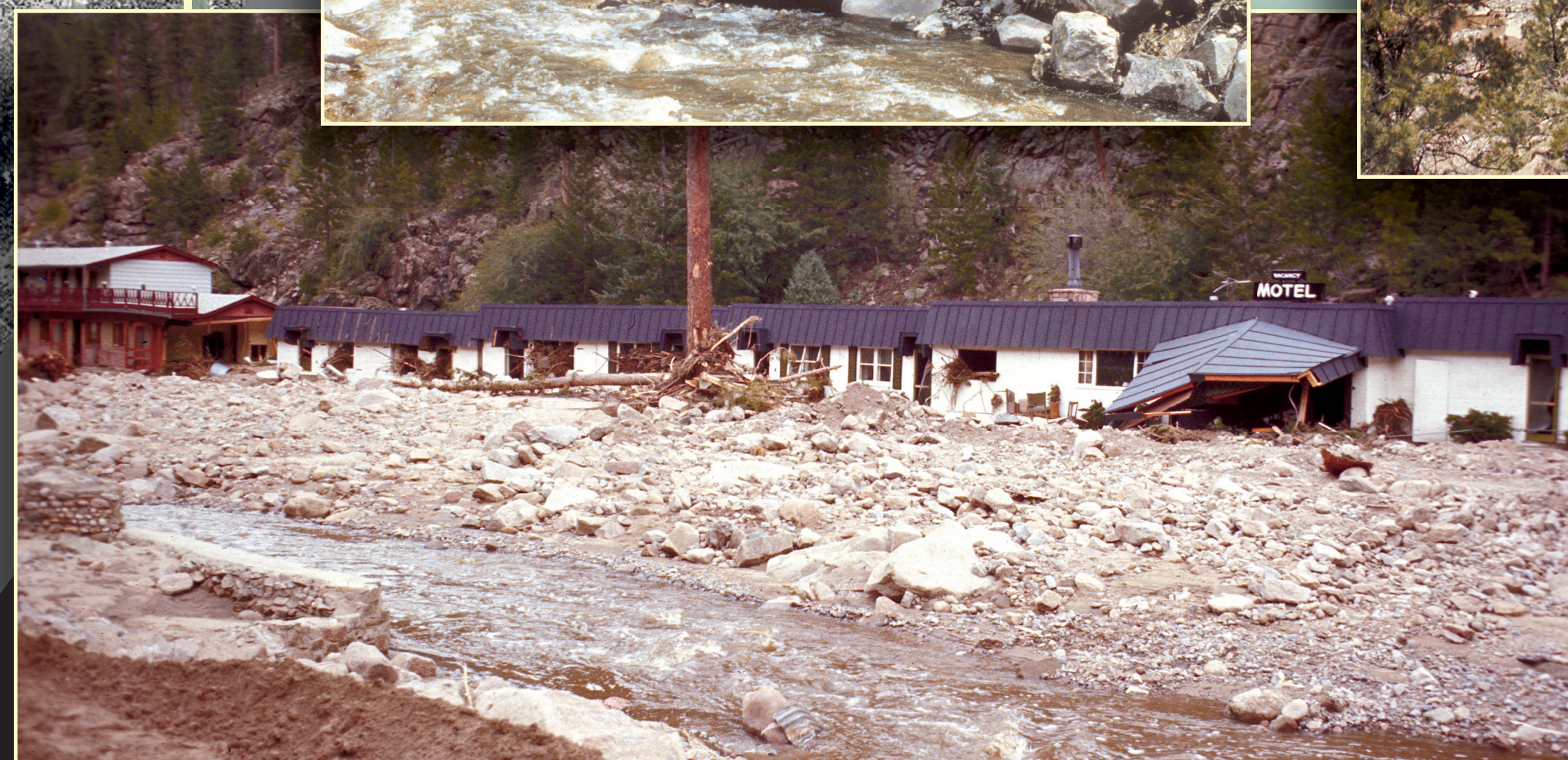
Downstream view of damaged Nihart Motel on the Big Thompson River near Glen Comfort.
