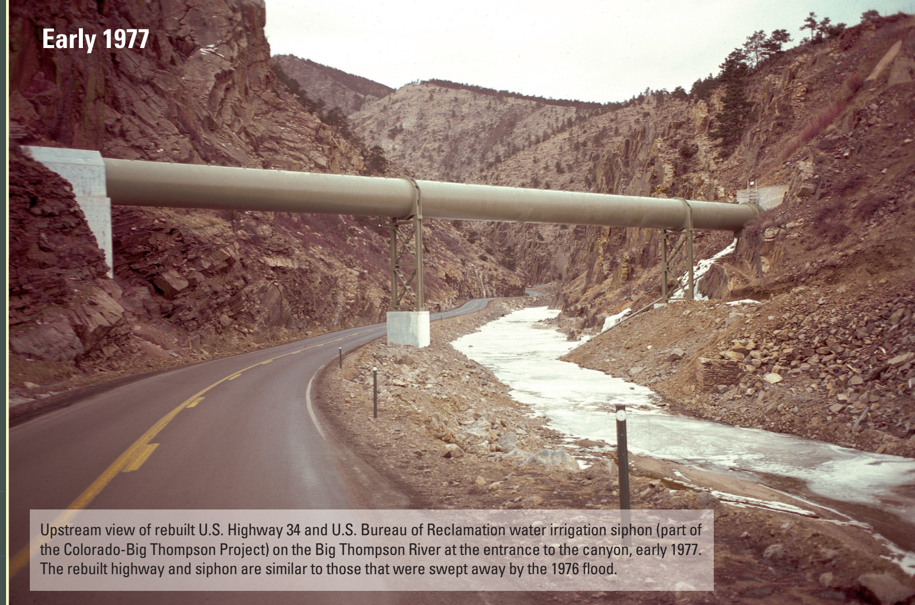
Upstream view of flood damage to U.S. Highway 34 and U.S. Bureau of Reclamation water irrigation siphon. In addition, a streamflow-gaging station was also swept away by the flood. Peak flood discharge was estimated to be 31,200 cubic feet per second in this area.
