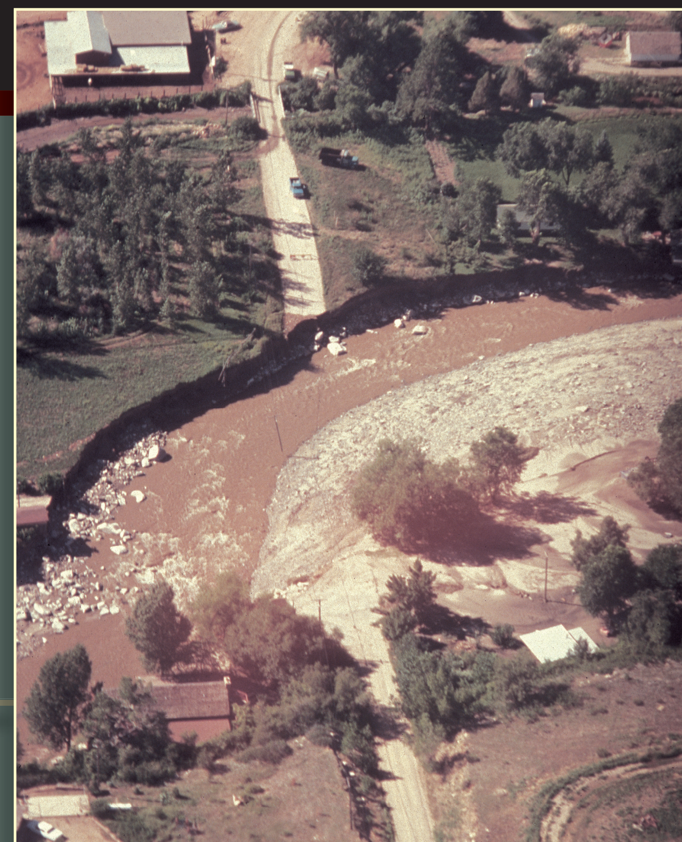
Bridge washed out on the Big Thompson River near Loveland as seen from a helicopter. Flow is from right to left.
