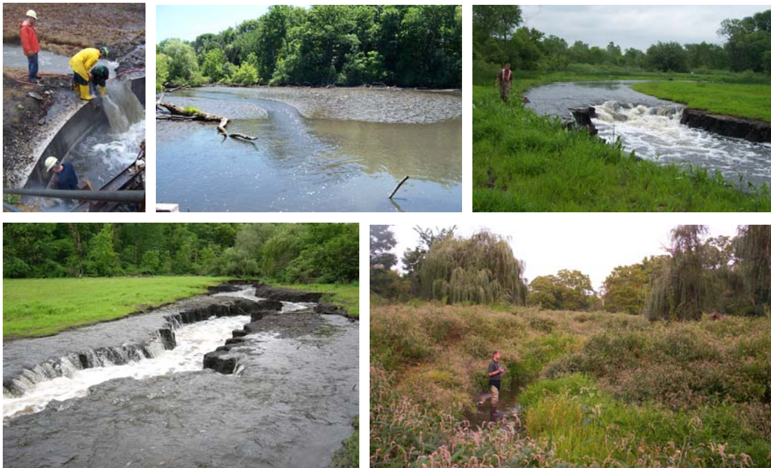
Figure 3. Top Left: Notching procedure during the fourth notch (November 2003). Top Middle: Dewatering of lake and channel formation after first notch (June 2003). Top Right and Bottom Left: Channel formation and headcut progression (May 2004). Bottom Right: Vegetated channel and riparian area (August 2005).
