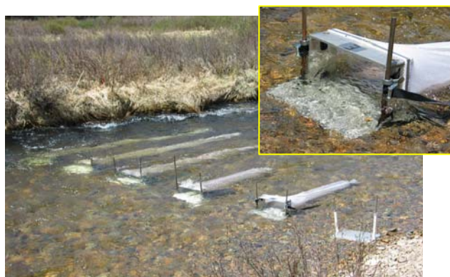
Figure 1 Bedload traps installed in a stream
