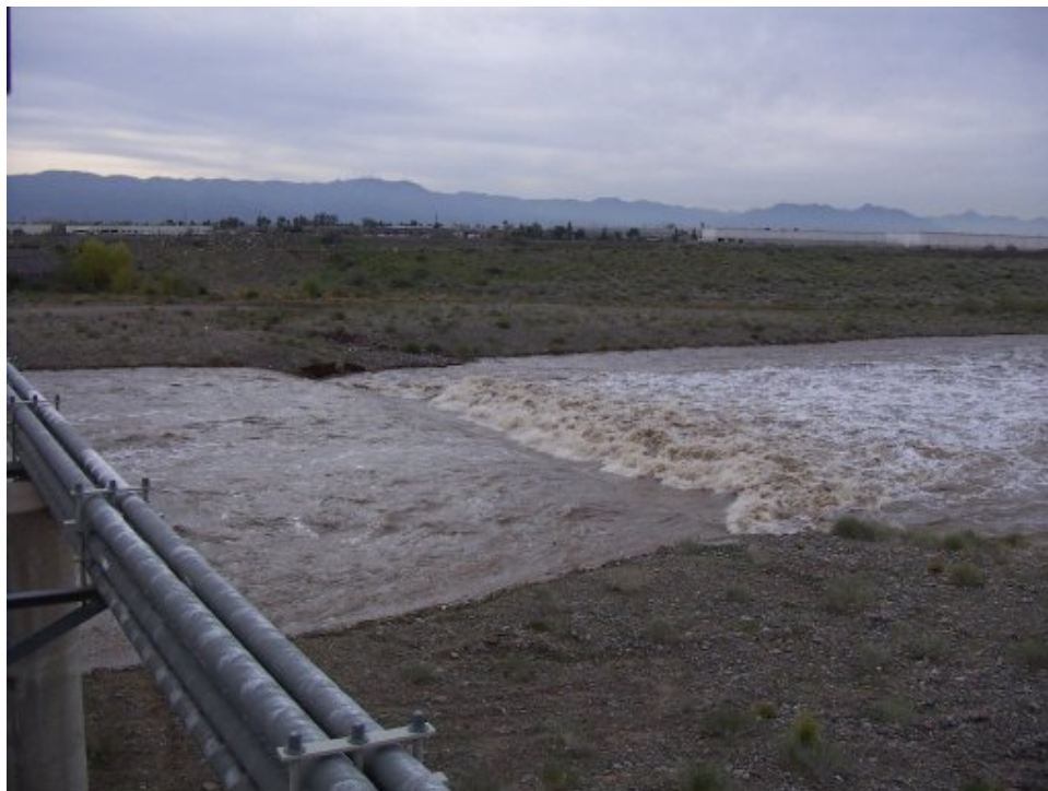
Figure 5 February 2005 flow at a grade control structure.
