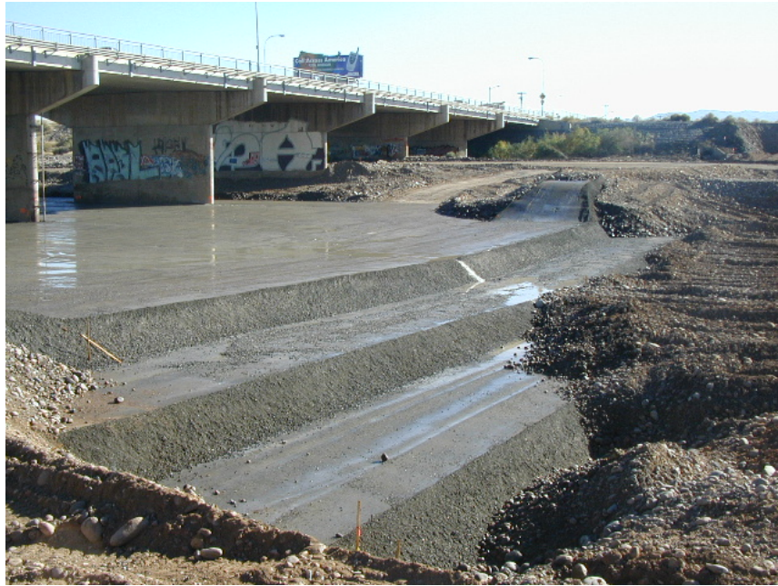
Figure 3 Grade control structure at the 24 th Street Bridge.
