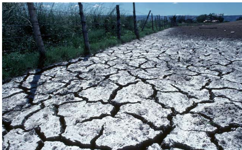
Figure 4 Desiccation Cracks in High Shrink-Swell Soils
