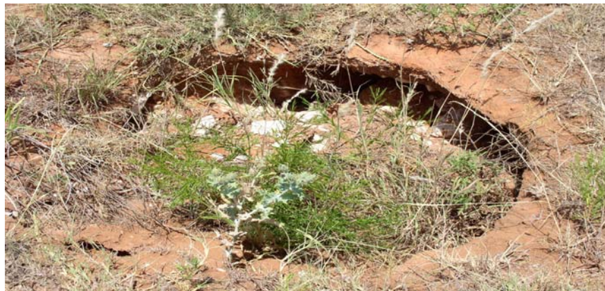
Figure 3 Sink Hole in Drained Sediment Pool, SW Oklahoma.
