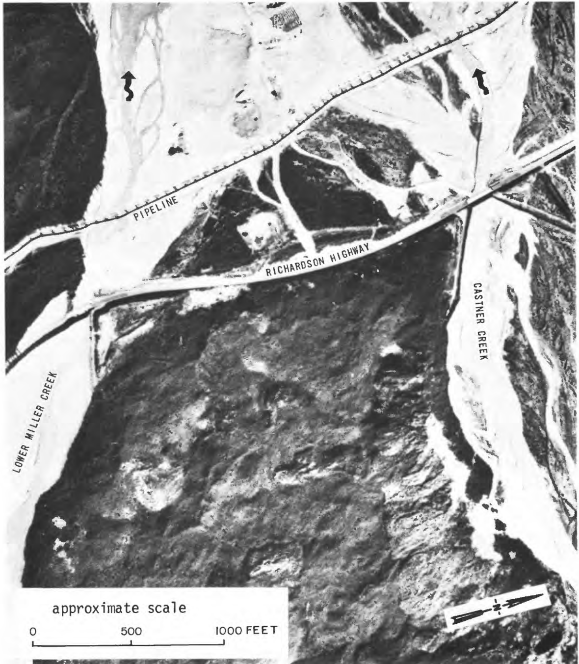
Figure 32. -- Castner and Lower Miller Creeks, July 29, 1977. AIR PHOTO TECH
