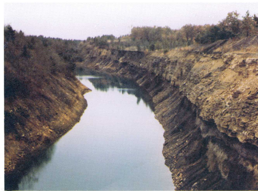
STRIP MINE RETENTION POND
