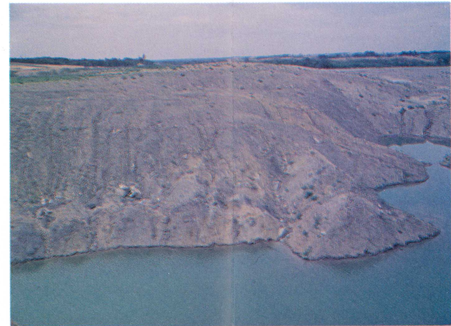
Figure 1.3-1 Erosion is accelerated at a partly reclaimed mine.
