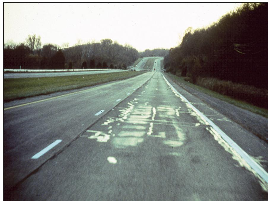
**Figure 5.** The oil on the surface of this road had been “stripped” from the aggregate because of the incompatible electrochemical properties of the aggregate and the bitumen binder. (Photo by D.W. Jahn)
