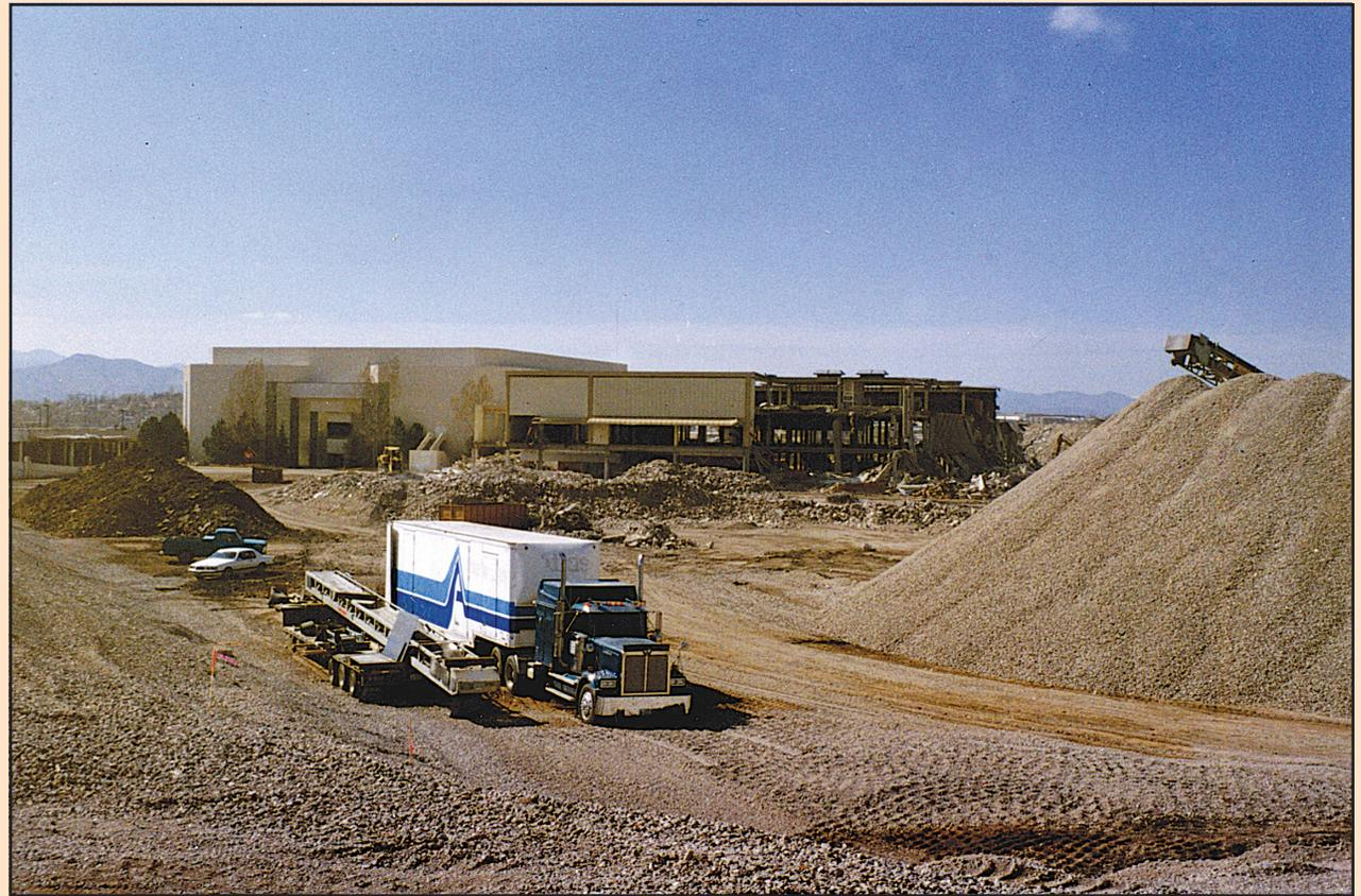
**Figure 3.** Some construction demolition material is recycled at the demolition site. (Photo by C.S. Mladnich, USGS)
