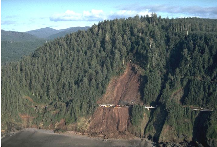
Figure 2: US 101 Cape Cove Landslide.
