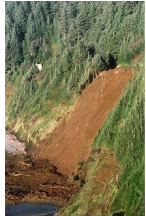
Fig 1: US 101 Cape Cove Landslide.
