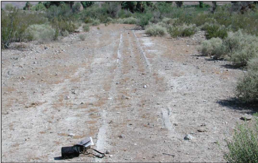
B. Former concrete irrigation ditch south of Cardy Lamb Swimming Pond that has been completely filled in with dirt.
