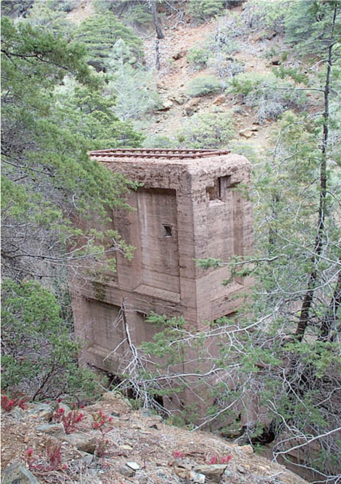
Figure 16. Central furnace at Research Mine with ore feed (upper right) and gas collectors.
