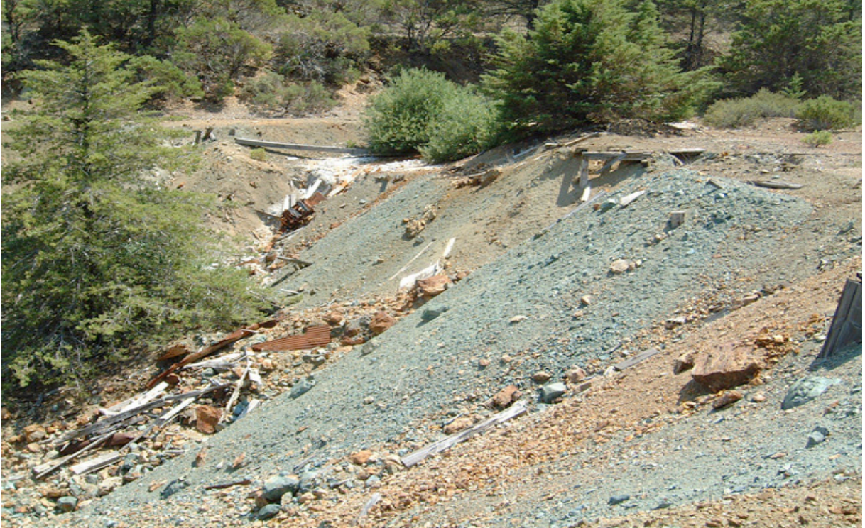
Figure 7. Mine drainage effluent channel in waste rock developed downstream from the Helen Mine.
