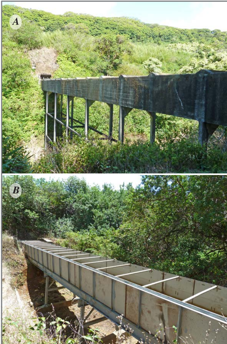
Figure 4. Photographs of two flumes that are part of the East Maui Irrigation diversion system, east Maui, Hawai'i. A , Concrete-lined flume along the Wailoa Ditch at 'Ōpana. B , Stainless-steel flume along the Lowrie Ditch near Kuiaha Gulch, also known as Labasan flume.
