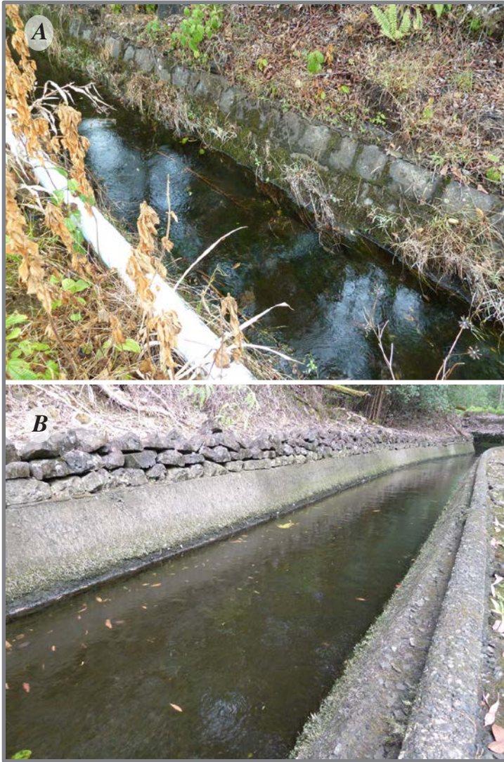
Figure 5. Photographs of two sections of the Ko'olau Ditch, East Maui Irrigation diversion system, east Maui, Hawai'i. A , Lined open-ditch section near Makapipi Stream with armored cut-stone walls and concrete bottom. B , Lined open-ditch section near Waiohue Stream with concrete walls and bottom.
