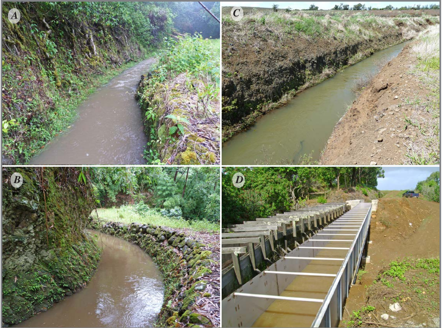
Figure 9. Photographs of Manuel Luis, Center, and Lowrie Ditches, East Maui Irrigation diversion system, east Maui, Hawai'i. A , Manuel Luis Ditch, unlined open-ditch section near Puohokamoa Stream. B , Center Ditch, unlined open-ditch section between Kōlea and Punalu'u Streams. C , Lowrie Ditch, unlined open-ditch section near Māliko Gulch. D , Lowrie Ditch, old wood flume and replacement stainless-steel flume near Pe'ahi Reservoir (photograph by Garret Hew, East Maui Irrigation Company).
