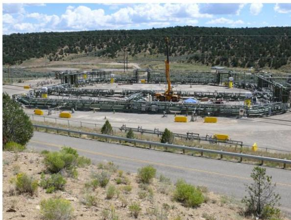
Photograph of freeze wall test by Shell Exploration and Production Company in the Piceance Basin.
