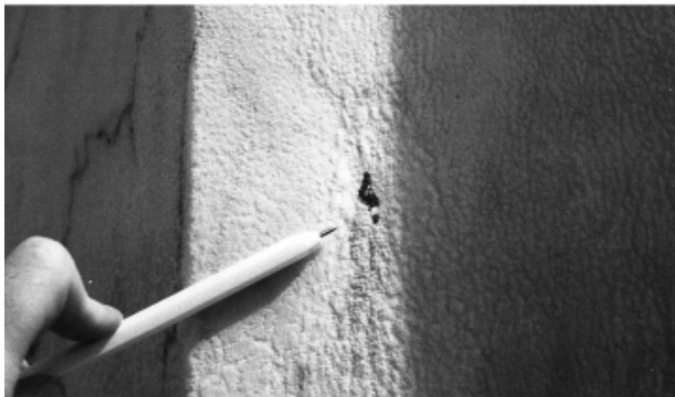
**Figure 13.** Sphalerite inclusion (dark grain) at the Lincoln Memorial occurs as an isolated grain with a rusty-brown surface. On weathered surfaces, sphalerite stands higher than the surrounding calcite.
