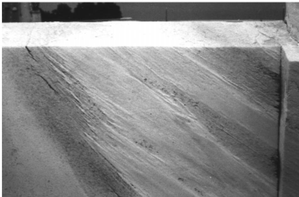
**Figure 14.** Differential wear on a cheneau piece along the roof at the Lincoln Memorial.
