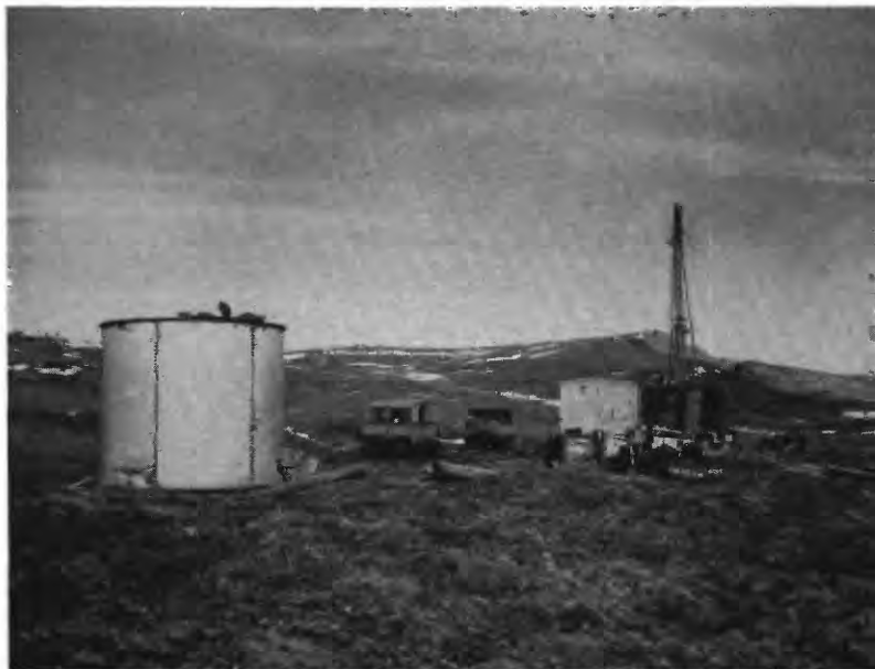
A. DRILLING RIG AT SITE OF UMIAT TEST WELL 4, JUNE 2, 1950
