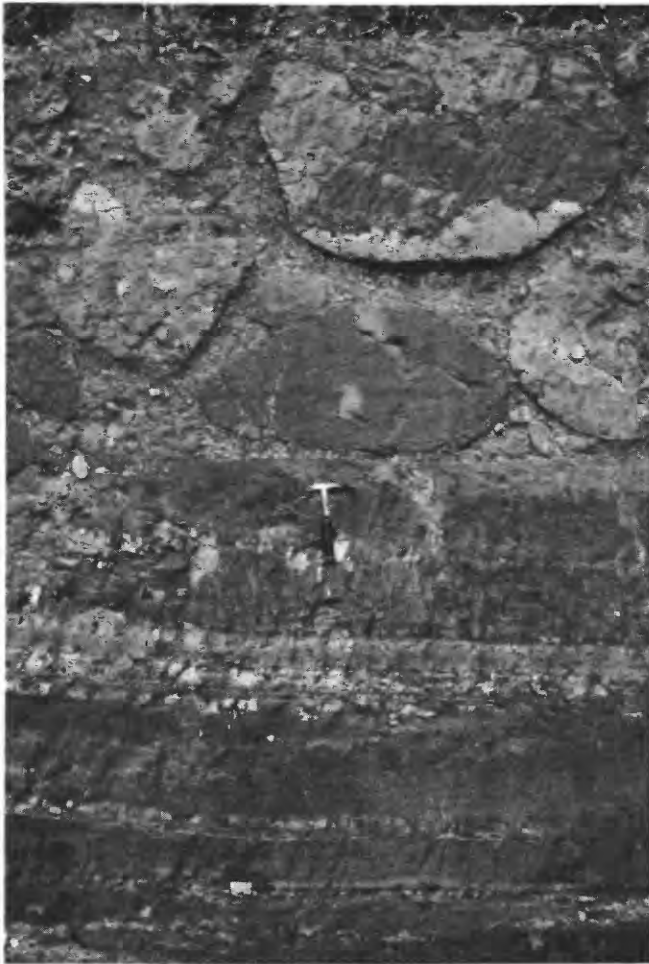
FIGURE 31.—Saprolite formed from rocks of the Nosoko Formation. Volcanic rock of the Nosoko Formation has completely changed to soft clayey material, but it still retains the structures of the original hard rock. The beds in the lower part of the picture were originally tuff. The large masses above were probably boulders in talus or slumped material that accumulated after the deposition of the tuff beds. This exposure is in a roadcut 1 kilometer southeast of Nosoko-ishi-zaki in the north part of the Nosoko peninsula. March 1956.
