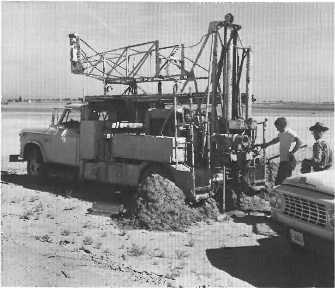
FIGURE 3.—Boring a test well with a power auger, 3\frac{1}{2} miles south of Somerton, Ariz.
