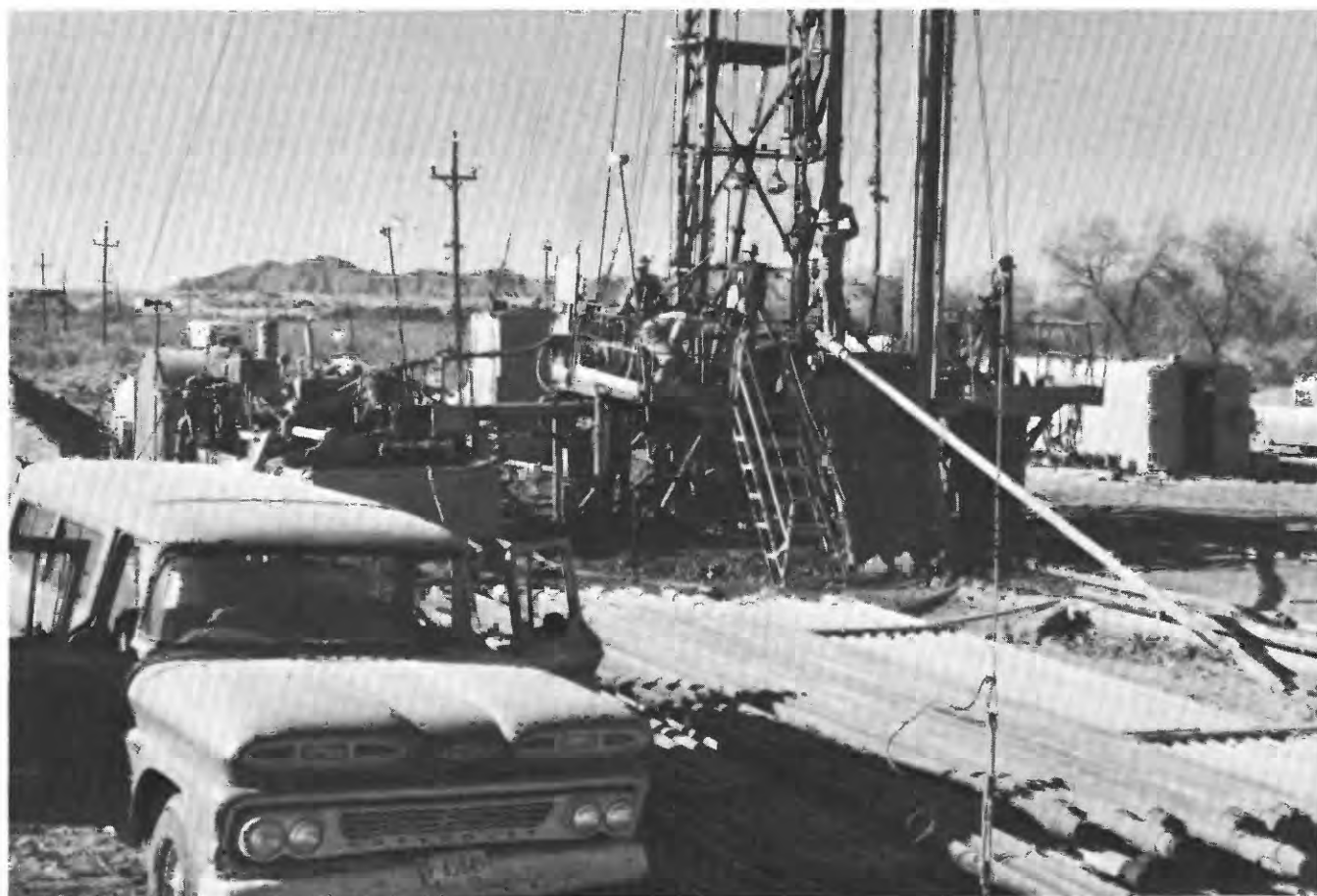
FIGURE 4.—Drilling of test well LCRP 26 with mud-rotary equipment 1½ miles west of Winterhaven, Calif.
