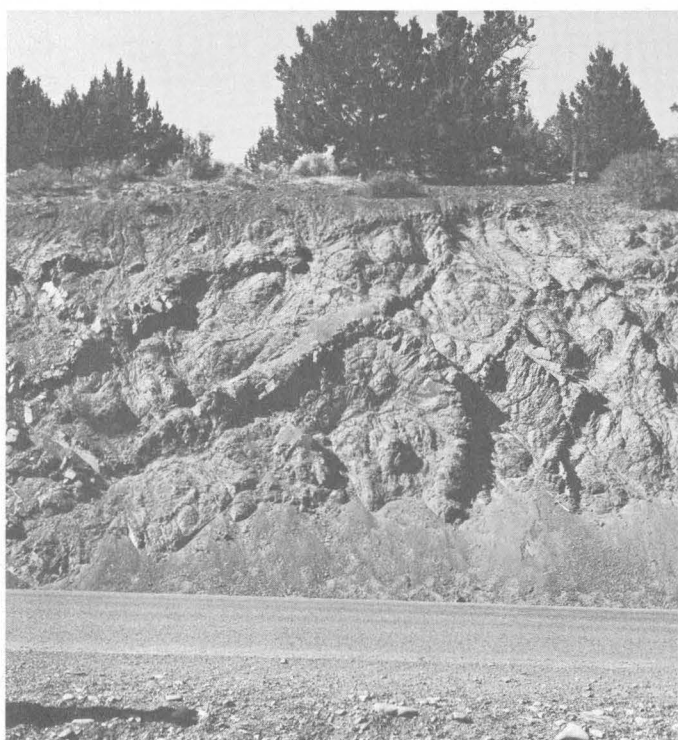
FIGURE 2.—Roadcuts on U.S. Highway 395, showing reticulate dikelike masses of unaltered andesite enclosing masses of soft friable andesite. Photograph at top shows mostly planar joint surfaces that occur on south side of highway near west end of exposure sequence. Photograph at bottom shows an exposure several hundred feet east on north side of highway where both planar and curved joint surfaces are common and are more widely spaced.
