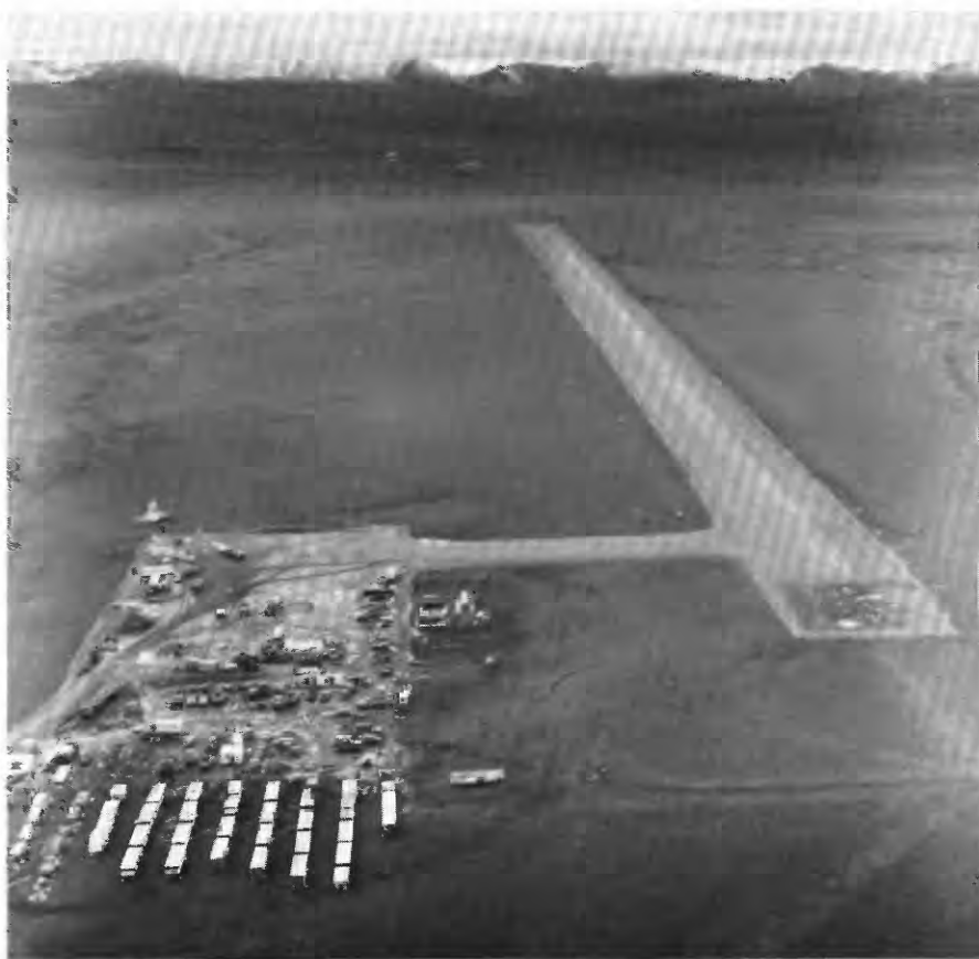
FIGURE 38.12.—Insulated all-season airstrip at Ivotuk, with parking apron and equipment storage area at left. Note wet overrun section at end of runway. View looking south taken in July 1979.
