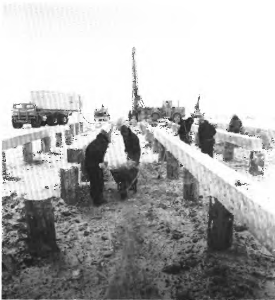
FIGURE 38.10.—Installing piling for drill rig at Tunalik. Rig in background is drilling conductor hole for well. View looking east taken in March 1978.
