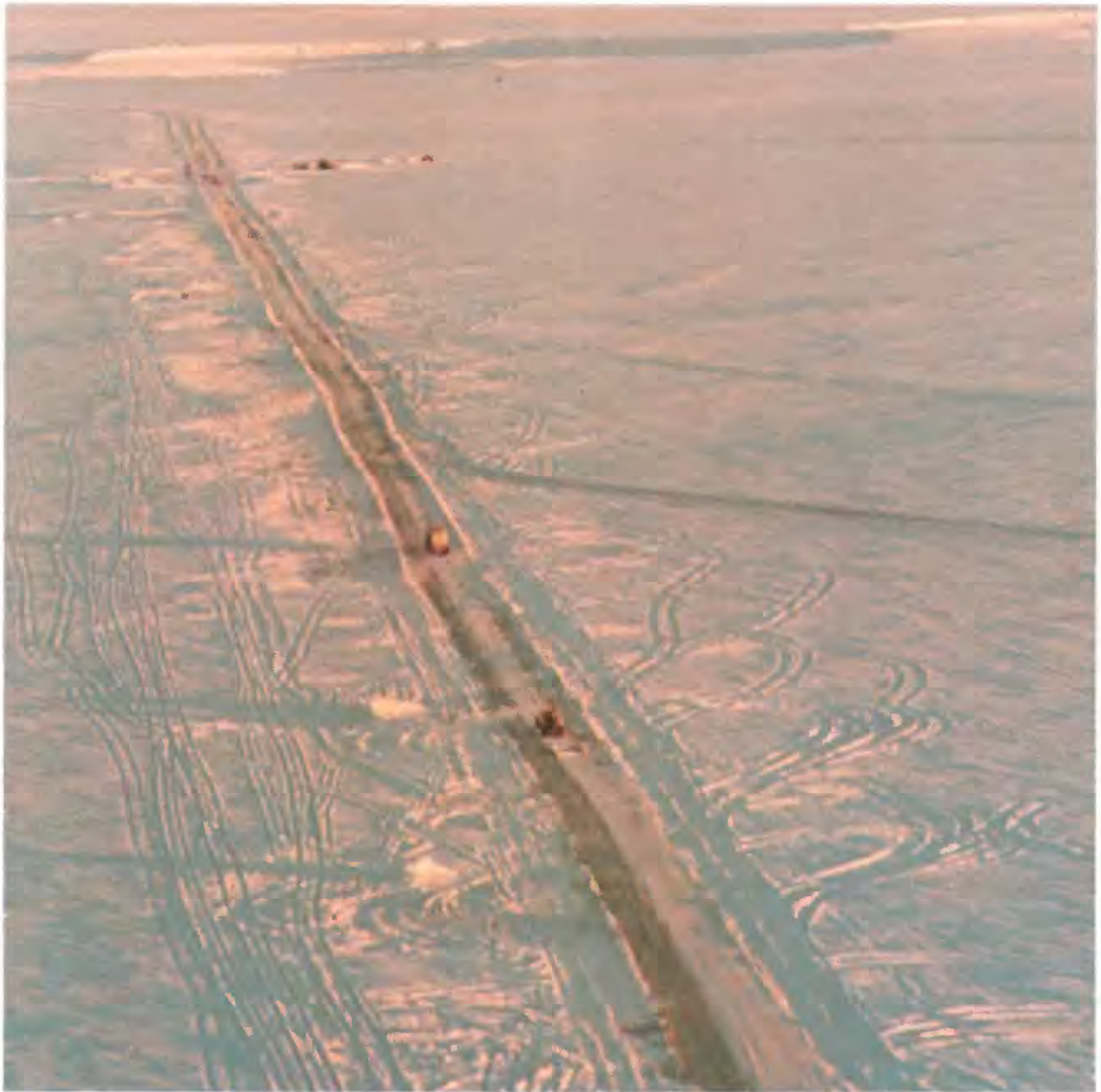
Aerial view of 59-km (37-mi) ice road from Kikiakrorak River delta to Inigok No. 1 well site, used to transport 70,000 m 3 (90,000 yd 3 or about 6,000 truckloads) of gravel to build the drill pad and airstrip. A total of 135,000 m 3 (35 million gallons) of water was required to form the ice road. Photograph by Jeep Johnson.
