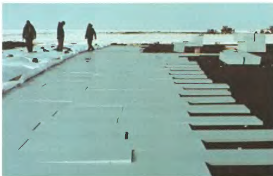
FIGURE 2.18.—Installing insulation on the Inigok runway, April 1978.
