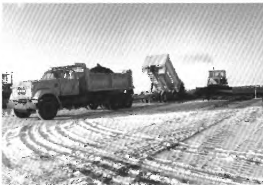
FIGURE 38.8.—Placing final lift of sand on subbase before placing insulation at Tunalik runway. Photograph taken in March 1978.
