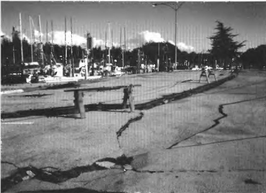
Figure 5.—Ground cracks at north end of Moss Landing Harbor District parking lot.
