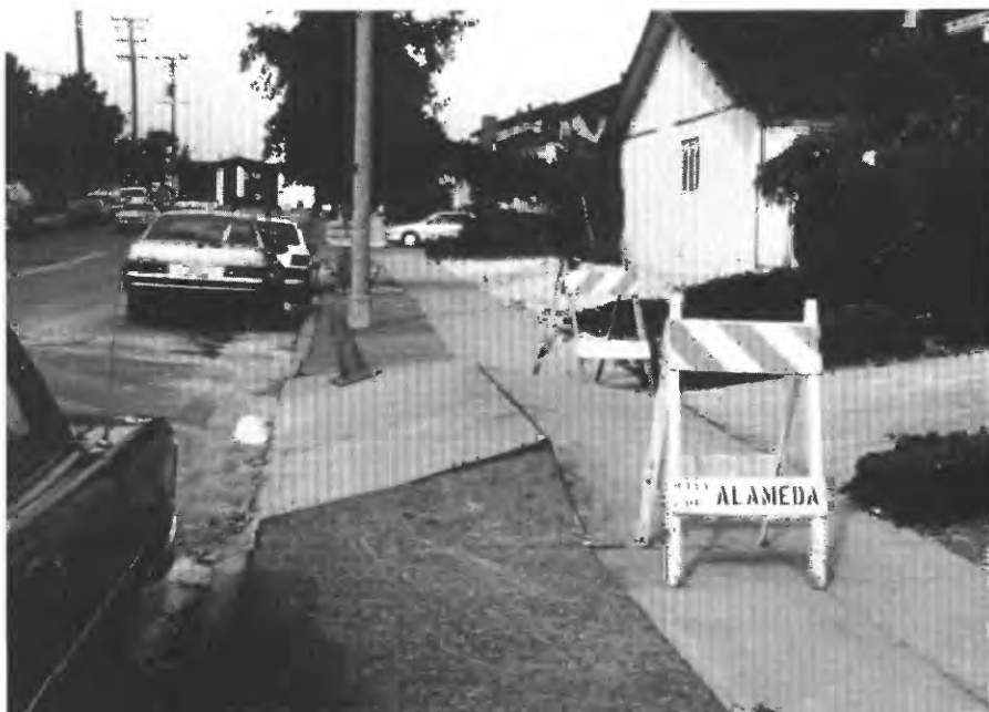
Figure 17.—Minor settlement and buckling of pavement at southwest edge of the Alameda (fig. 1).
