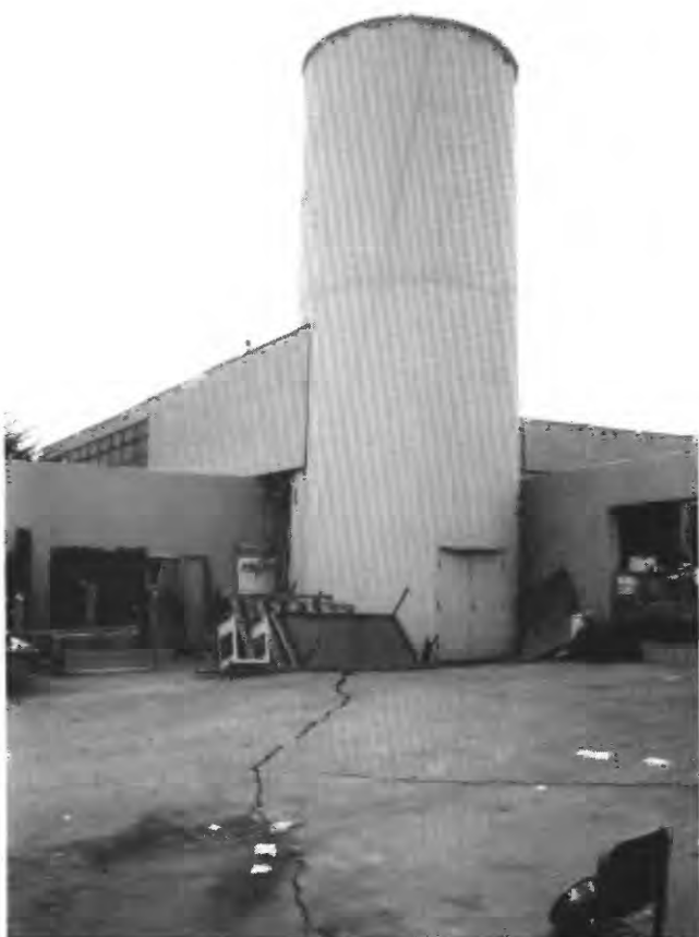
Figure 16.—Cracks in corporation-yard pavement of Moss Landing Marine Laboratory (fig. 11). Seawater-storage tank in background settled differentially 2 to 3 in.
