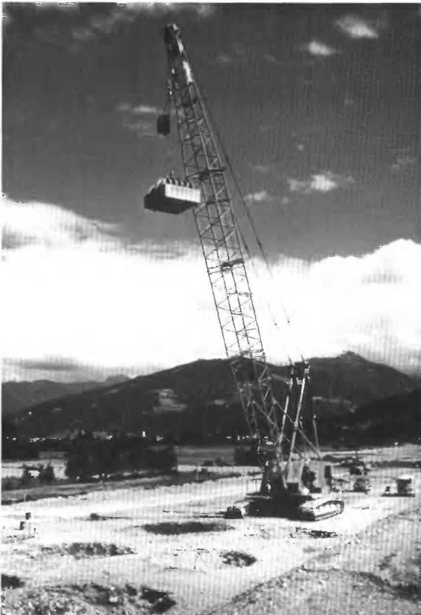
Figure 3.—Dynamic deep compaction in operation.
