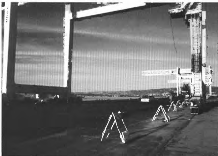
Figure 11.—Wharf of Port of Oakland's Marine Container Terminal at Seventh Street (viewed from Berth 37), showing shipping-container cranes, damaged pavement, and extruded sand.
