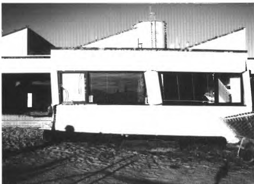
Figure 13.—Racking of southern building at southeast corner of Moss Landing Marine Laboratory (fig. 11).
