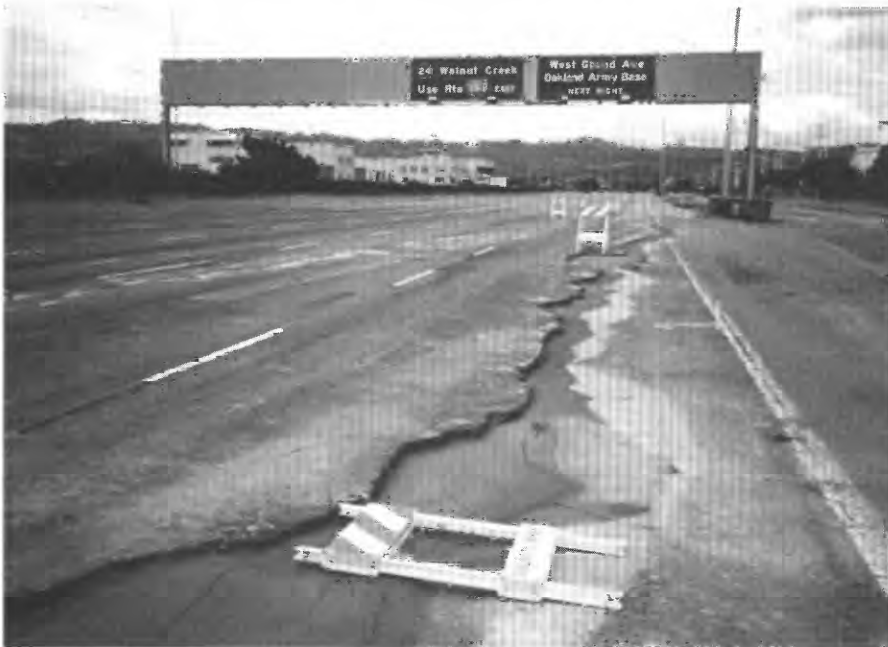
Figure 6.—Fissure in pavement caused by settlement in rightmost eastbound lane of Interstate Highway 80 west of San Francisco-Oakland Bay Bridge Toll Plaza administration building (visible in distance).
