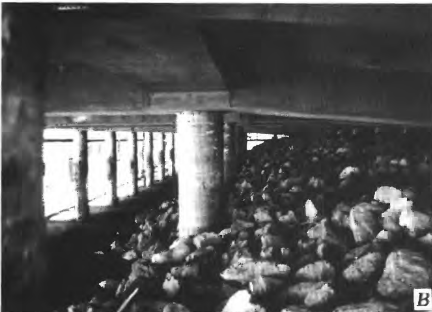
Figure 21.—Appearance of Monterey Bay Aquarium Research Institute pier 3 days after earthquake. A, South side of pier. B, Under-side of concrete deck.
