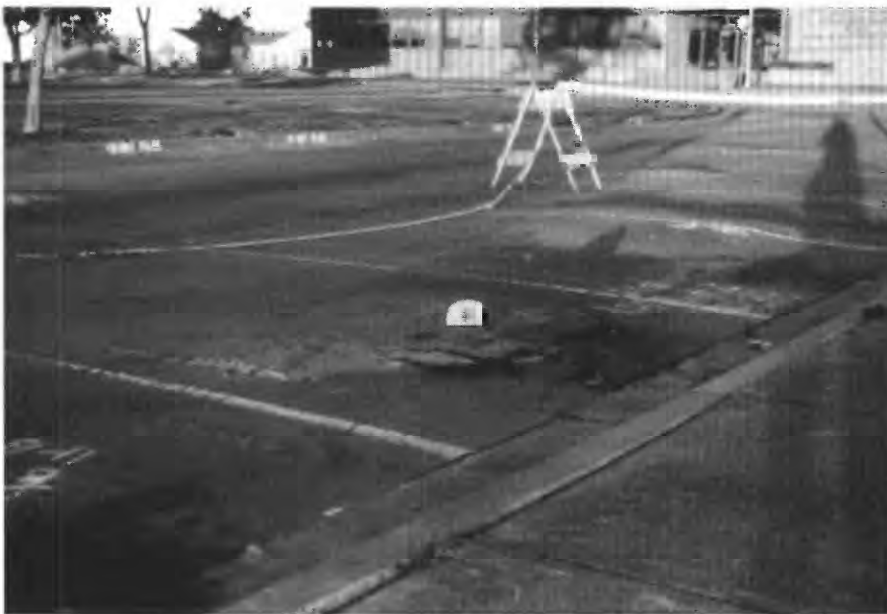
Figure 6.—Differential settlement (approx 90 mm) on Treasure Island where piles erupted through pavement in parking lot near Building 450 (loc. 28, fig. 4).
