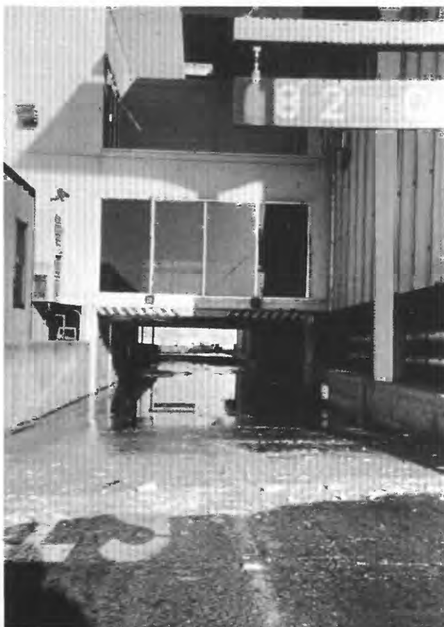
Figure 25.—Below-grade tramway, filled with as much as 1.8 m of extruded sand, at Oakland International Airport Terminal Building. Photograph courtesy of B.A. Vallergera.
