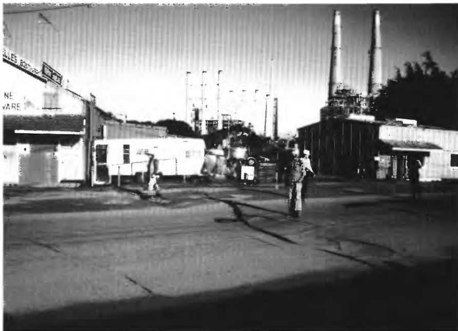
Figure 7.—Settlement across Sandholdt Road near north end of Moss Landing spit (see fig. 2 for locations).
