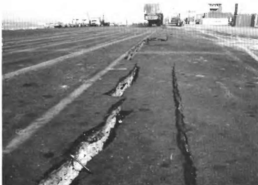
Figure 12.—Closeup of damaged pavement near boreholes POO7-5 and POO7-6 at Port of Oakland Berths 36 and 37 (see fig. 5 for locations), showing differential settlement, open fissures, and lateral spreading.
