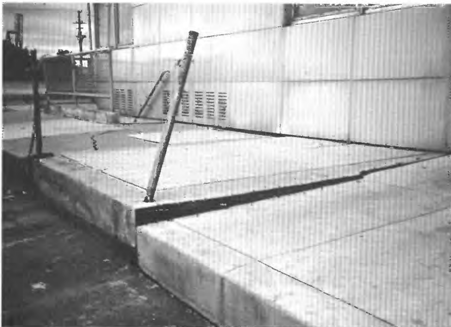
Figure 7.—Settlement at the east side of the San Francisco-Oakland Bay Bridge Toll Plaza administration building.
