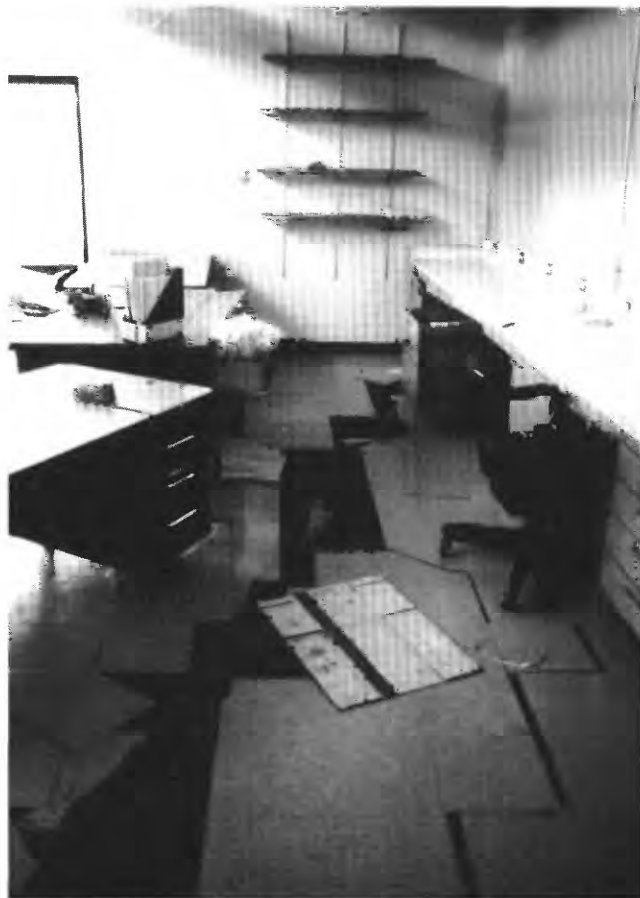
Figure 14.—Cracks in concrete floor in southern building of Moss Landing Marine Laboratory (fig. 11).
