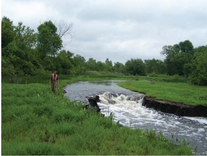
Figure 5. Diagram of a nickpoint (modified from Schumm and others, 1984) (top), and example of nickpoint progression after gradual removal of Brewster Creek dam near St. Charles, Illinois (bottom).
