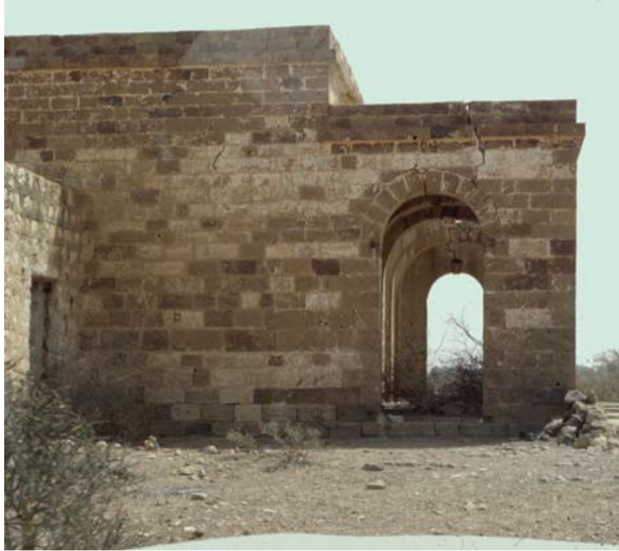
Figure 7. Photograph of the Band Virah chauki (police station), Pakistan. Broken arches and missing stones are attributed to earthquake damage after 1947. The building is visible in the background of figure 6, and the approximate location of the area is shown in figure 2 by the x. Photograph by W.F. Outerbridge (USGS, 1985).
