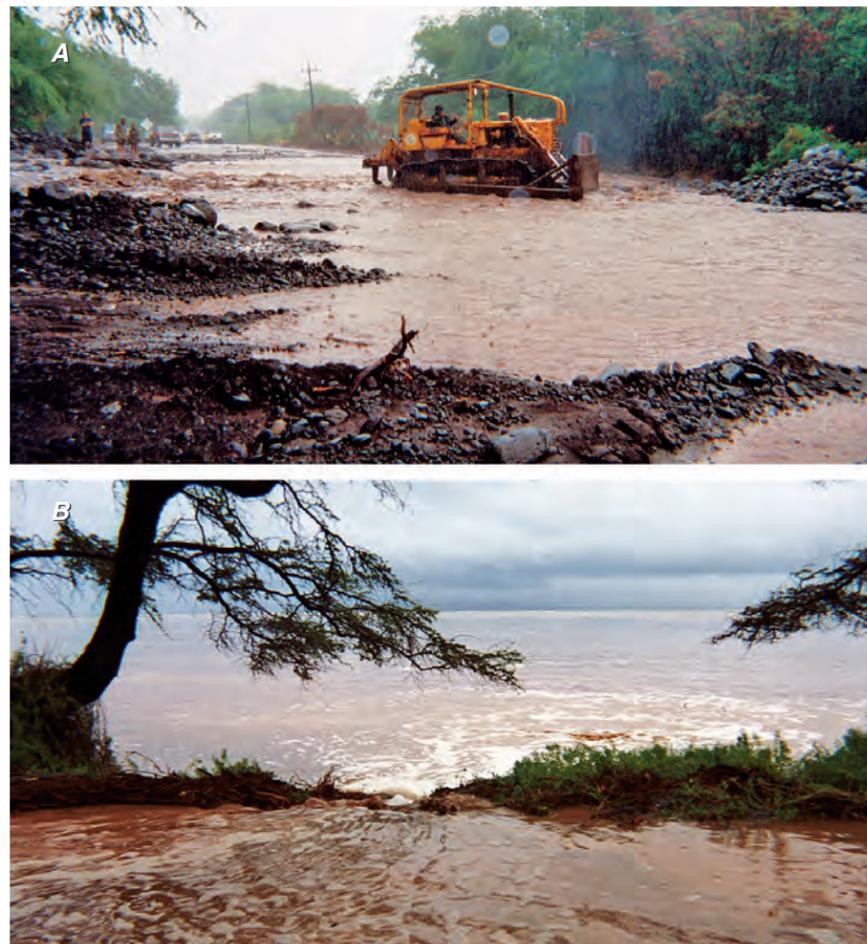
**Figure 4.** Sediment transport and deposition resulting from the November 2001 storm on Moloka'i. *A*, Highway 450 near mile marker 7, showing sediment deposits on roadbed. Closures such as this are common along this stretch of road and typically occur about once a winter. *B*, Overland flow of sediment across Highway 450 and onto the reef flat near mile marker 6.
