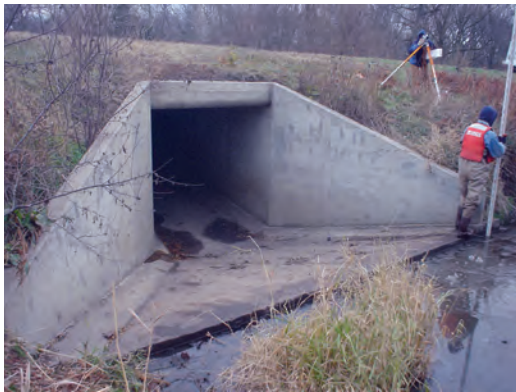
Grade control on the upstream side of Southwest 27th Street
