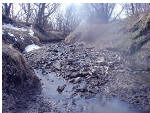
Piled rock at a hiking-trail crossing that is providing grade control
