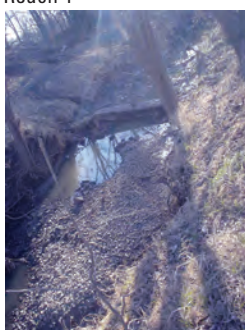
Remnants of an abandoned low-water crossing that is now providing marginal grade control
