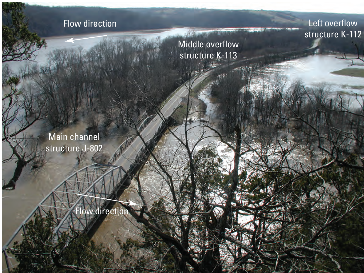
Figure 1. State Highway 17 crossing the Gasconade River near Waynesville, Missouri, as viewed from a bluff on the downstream right bank facing west-south-west on March 21, 2008, one day after the peak for a flood on March 20, 2008.
