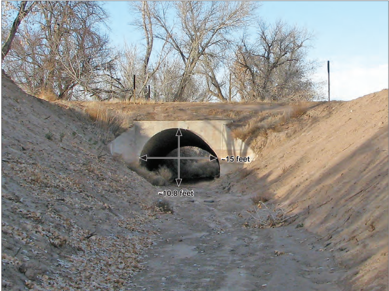
Figure 12. Main Street culvert in Bull Creek, Utah.
