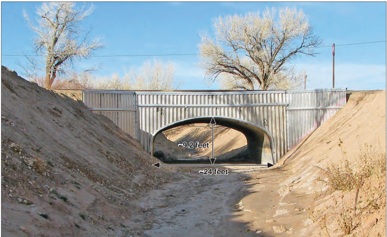
Figure 11. 100 South Bridge in Bull Creek, Utah.
