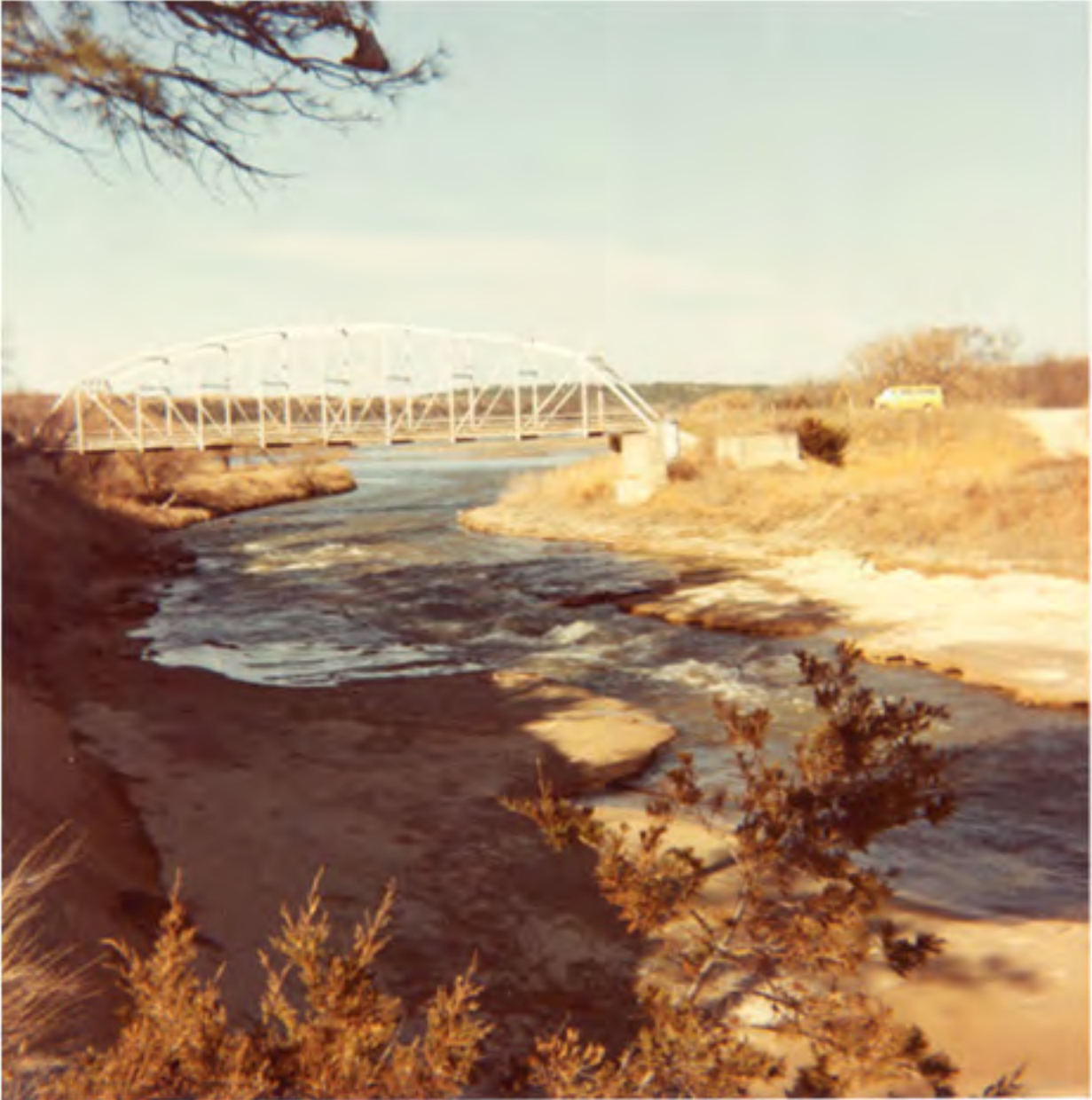
Figure 1-4. Photograph of the Niobrara River near Norden streamflow-gaging station reach. Photo was taken looking upstream from the right river bank. The gage house can be seen on the left river bank (right side of photo), just downstream from the bridge. Discharge measurements were made by both wading and using the bridge. However, only bridge measurements were used for the hydraulic geometry relation. The bedrock notch is now located several meters upstream from the bridge. (USGS file photograph)
