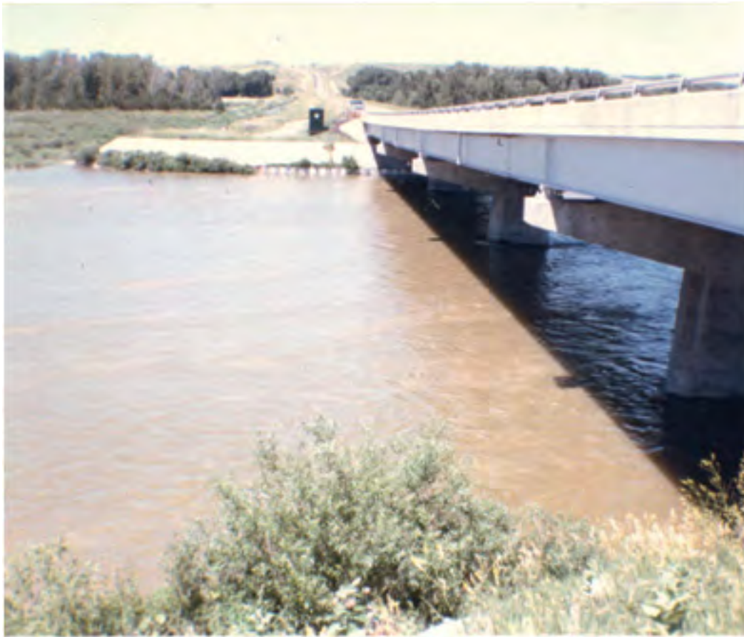
Figure 1-5. Photograph of the Niobrara River near Mariaville streamflow-gaging station reach. Photo was taken from the left river bank looking toward the right river bank. Gage house can be seen on opposite side of river. Flow is from right to left. Discharge measurements were made by both wading and using the bridge. However, only bridge measurements were used for the hydraulic geometry relation. (Photograph taken by Mark Nelson, Nebraska Department of Natural Resources)
