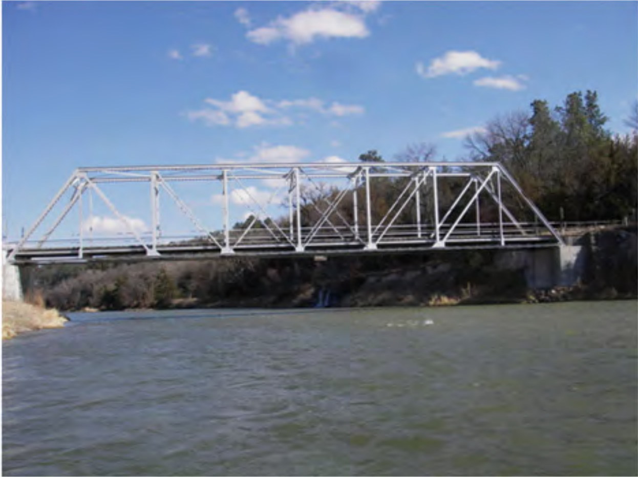
Figure 1-3. Photograph of the Niobrara River near Sparks streamflow-gaging station reach. Photo was taken looking downstream. The gage house is on the left bank, immediately downstream from the bridge. Most discharge measurements were made by wading downstream from the bridge. High-flow measurements are made from the bridge. (Photograph taken by Ronald Zelt, USGS).
