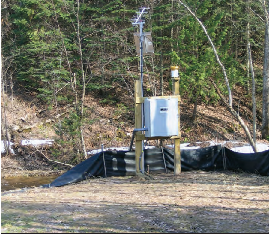
Figure 13. U.S. Geological Survey streamgage at Gomanche Creek at Indian Road (04043140). (Photograph by T.L. Weaver, U.S. Geological Survey)
