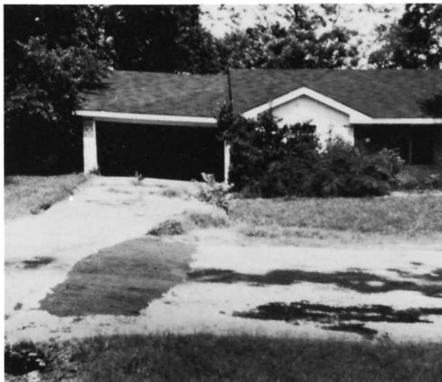
Figure 2. House damaged by a fault in northwest Houston. Fault has deformed garage and has required patch in road.
