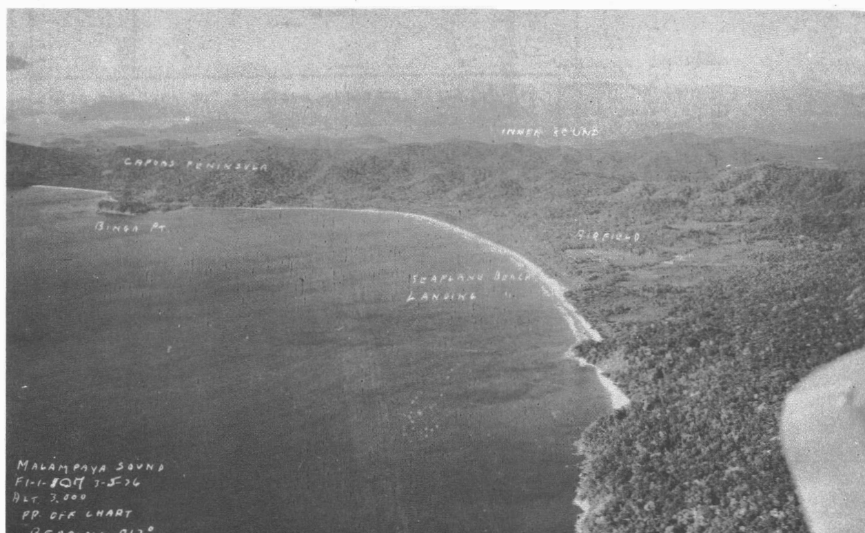
Airfield site southeast Binga Point; view to northeast. (ONI 62813)
