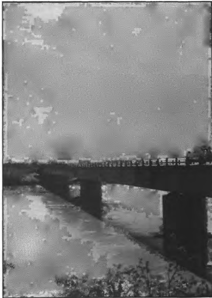
Figure 4. Bridge 331 on the Copper River Highway in 1991.
