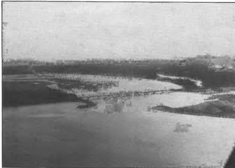
Figure 22B. Bridge 342 on the Copper River Highway, looking downstream; top, September 1991; bottom, September 1992.
