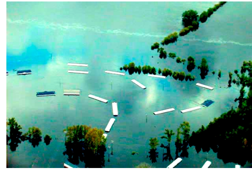
Flooded mobile home park along the Tar River
