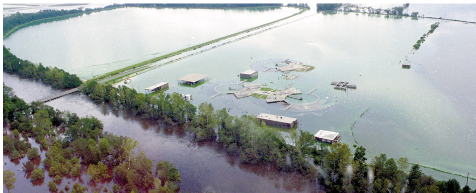
Wastewater-treatment plant in Goldsboro, N.C.
