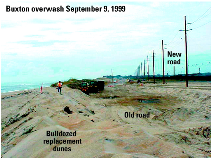
Figure 25. Former location of N.C. Highway 12 near Buxton and replacement dunes.
