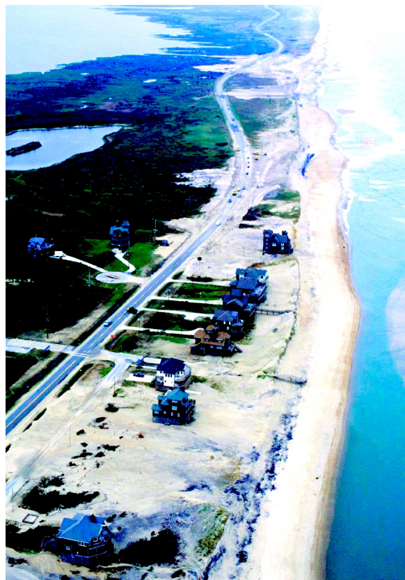
Extensive dune erosion resulting from Hurricane Dennis, northern Outer Banks
