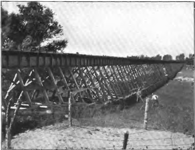
B. WILSON CANAL FLUME, WEBER COUNTY, UTAH.
