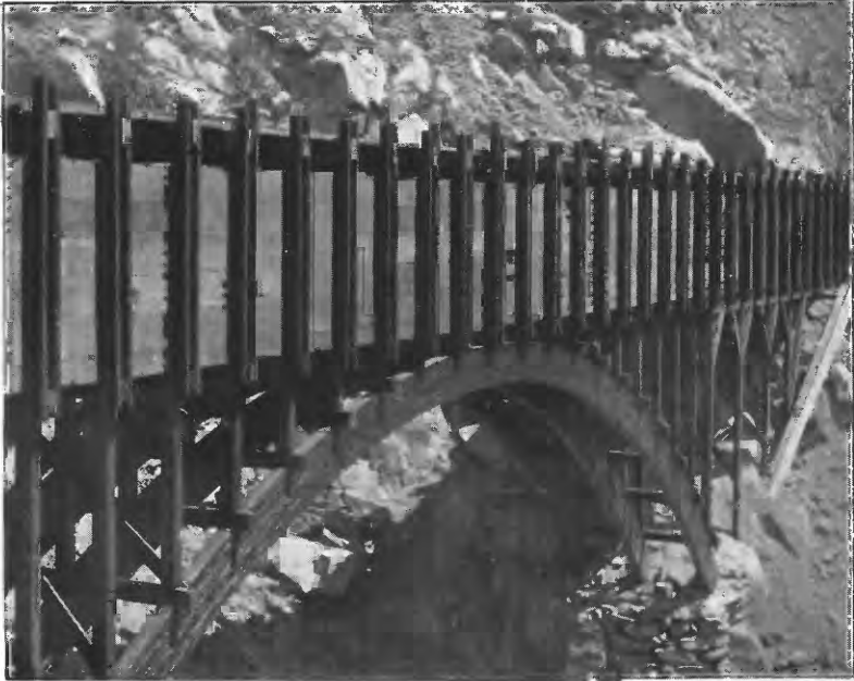
A. FLUME OF KERN VALLEY POWER DEVELOPMENT WORKS, CALIFORNIA.
