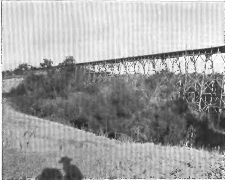
B. FLUME AT SANGER, CALIFORNIA.
