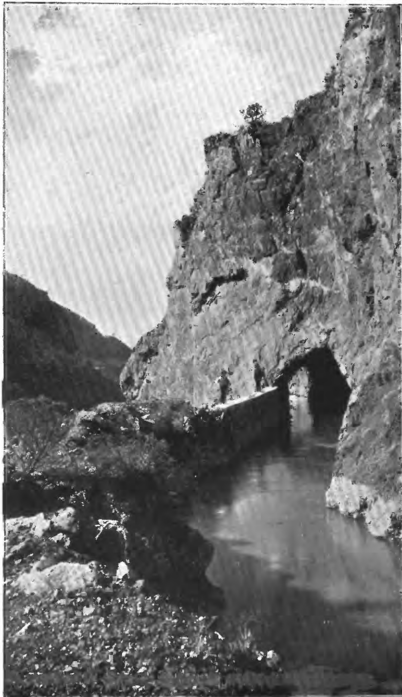
TUNNEL OF BEAR RIVER CANAL, UTAH.
