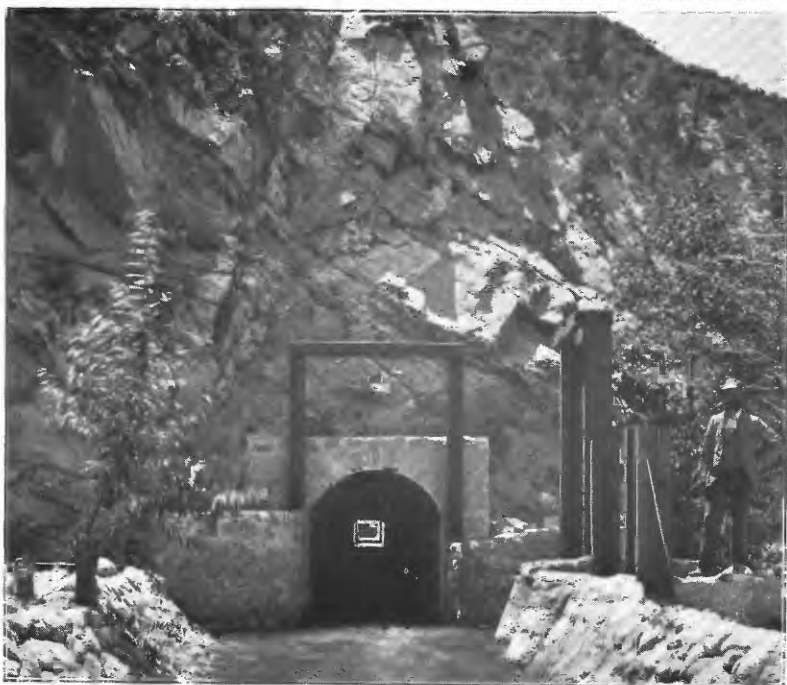
A. TEMPORARY HEADWORKS OF SANTA ANA CANAL, CALIFORNIA.
