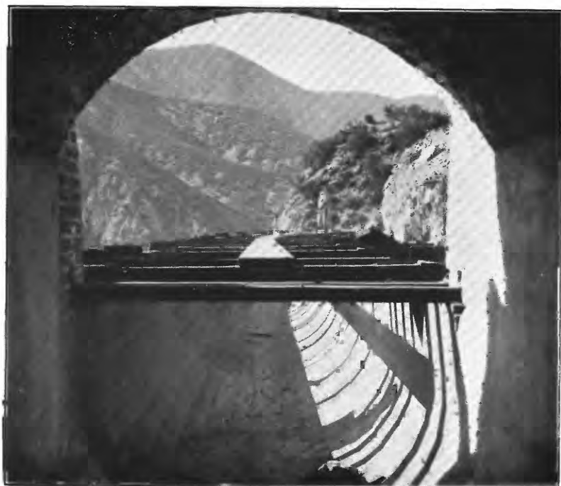
B. CONNECTION BETWEEN TUNNEL AND FLUME OF SANTA ANA CANAL, CALIFORNIA.
