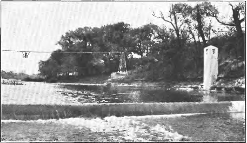
A. ARTIFICIAL CONTROL, RECORDER HOUSE, AND MEASURING CABLE ON OLEN-TANGY RIVER, DELAWARE, OHIO.
