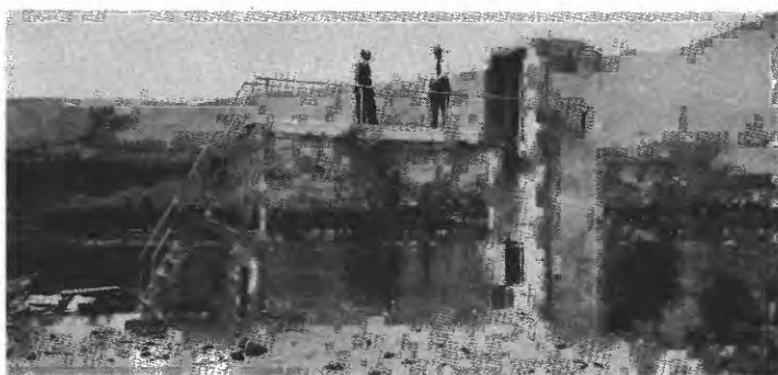
B. COLUMBIA RIVER NEAR THE DALLES, OREG. Gage shelter and stilling well.
