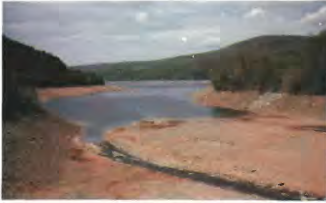
Figure 12. Pepacton Reservoir, New York, on May 19, 1985. Reservoir storage on that day was 263,040 acre-feet (85.7 billion gallons), which was about 61 percent of capacity; water-level elevation was 1,246.65 feet above sea level. By mid-September just before Hurricane Gloria, the reservoir level had dropped to 1,217.8 feet and the reservoir storage was 153,440 acre-feet (50.0 billion gallons), which was 36 percent of capacity. The spillway level (treeline on photograph) is 1,280 feet. (Photograph courtesy of Alison Peck Smith, The River Reporter , Narrowsburg, N.Y.)
