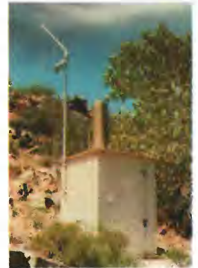
Figure 77. U.S. Geological Survey hydrologic-data station at Turkey Creek near Cleator, Ariz., equipped with a Data-Collection Platform aimed at one of the Geostationary Operational Environmental Satellites. (Photograph by John W. H. Blee, U.S. Geological Survey.)
