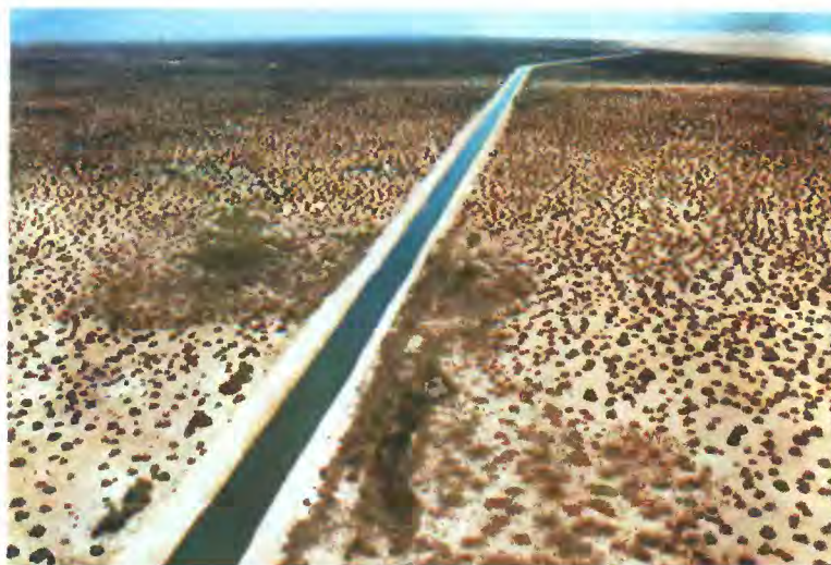
Figure 86. Coachella Canal in southern California. The heavy vegetation near the canal in the foreground indicates an area of leakage from this unlined section, which has been lined since this picture was taken. Similar water losses occur from facilities owned by the Imperial Irrigation District. (Photograph courtesy of U.S. Bureau of Reclamation.)
