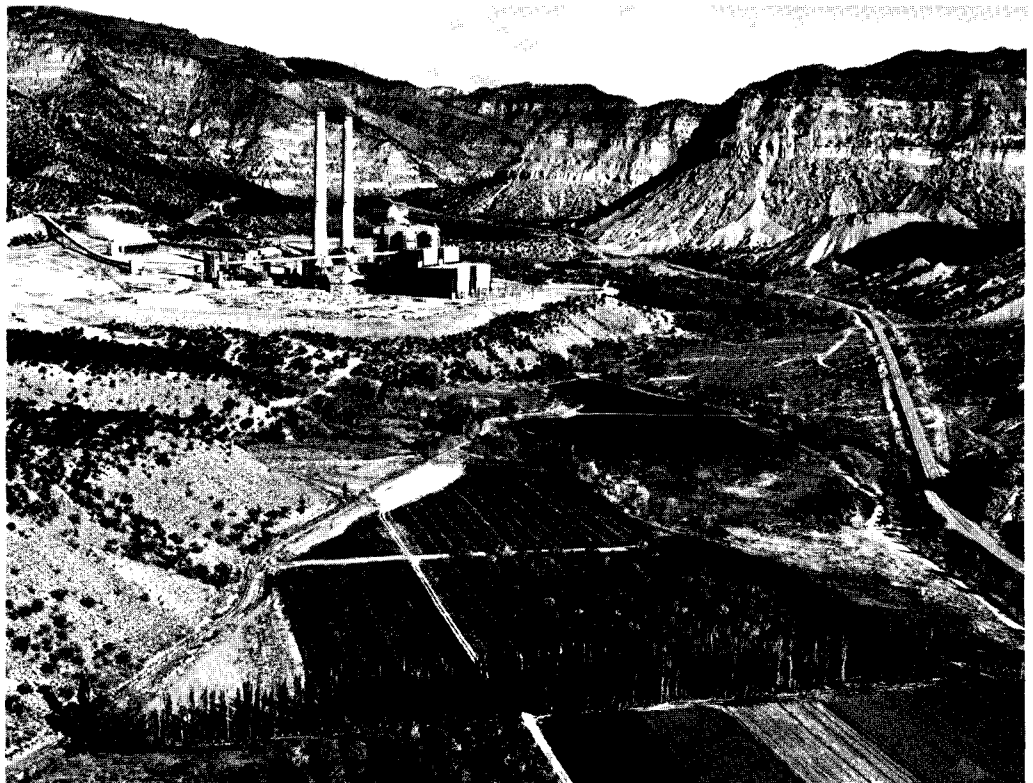
Figure 85. Huntington Unit of the Utah Power and Light Company. Water formerly used for irrigation of lands similar to those in the foreground has been transferred for use by the coal-fired thermoelectric powerplant. Most of the water is used for evaporative cooling; note the water vapor rising from the cooling tower. (Photograph courtesy of Utah Power & Light Co., May 1978.)
