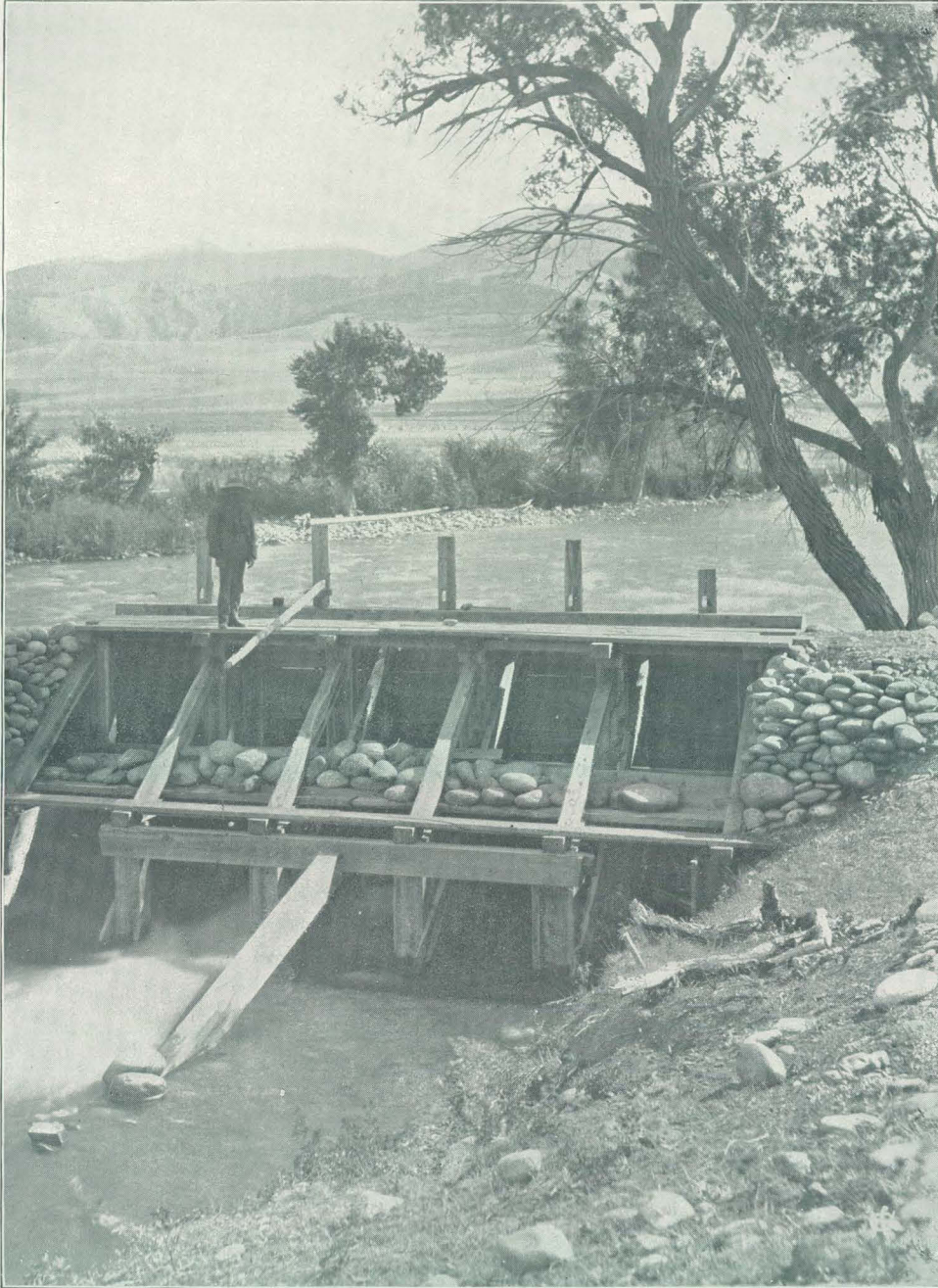
HEAD GATE OF CANAL OF THE WEST GALLATIN IRRIGATION COMPANY, GALLATIN COUNTY, MONTANA.
