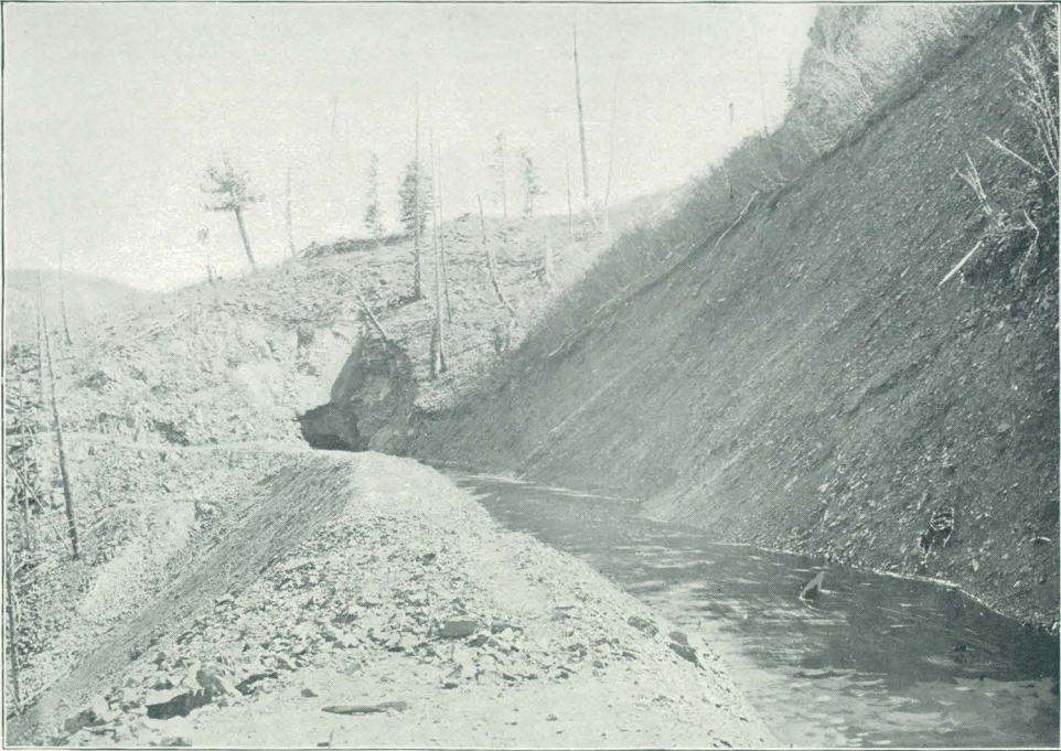
A. SKY-LINE DITCH—DIVERTING WATER FROM LARAMIE RIVER TO CACHE LA POUFRE RIVER.
