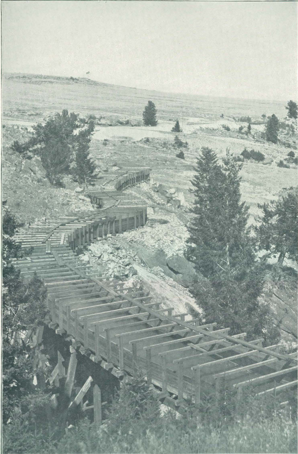
FLUME AND TRESTLE ACROSS ROCKY CANYON, MONTANA.
