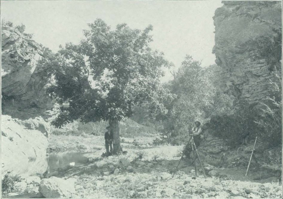
A. DAM SITE OF SMALL RESERVOIR ON HORSESHOE CREEK, WYOMING.
