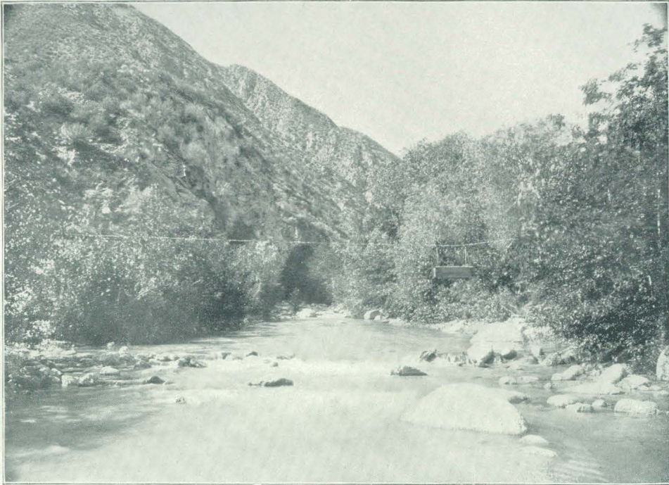
1. GAGING STATION ON SANTA ANA RIVER AT WARMSPRINGS, CALIFORNIA.
