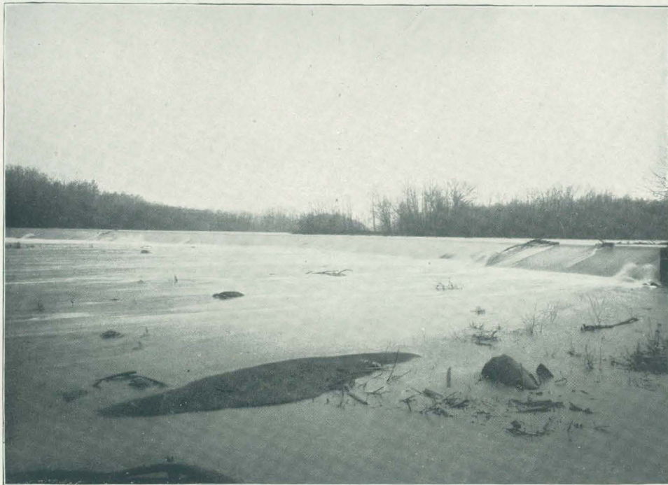
A. DAM ACROSS DEEP RIVER NEAR LOCKVILLE, NORTH CAROLINA.
