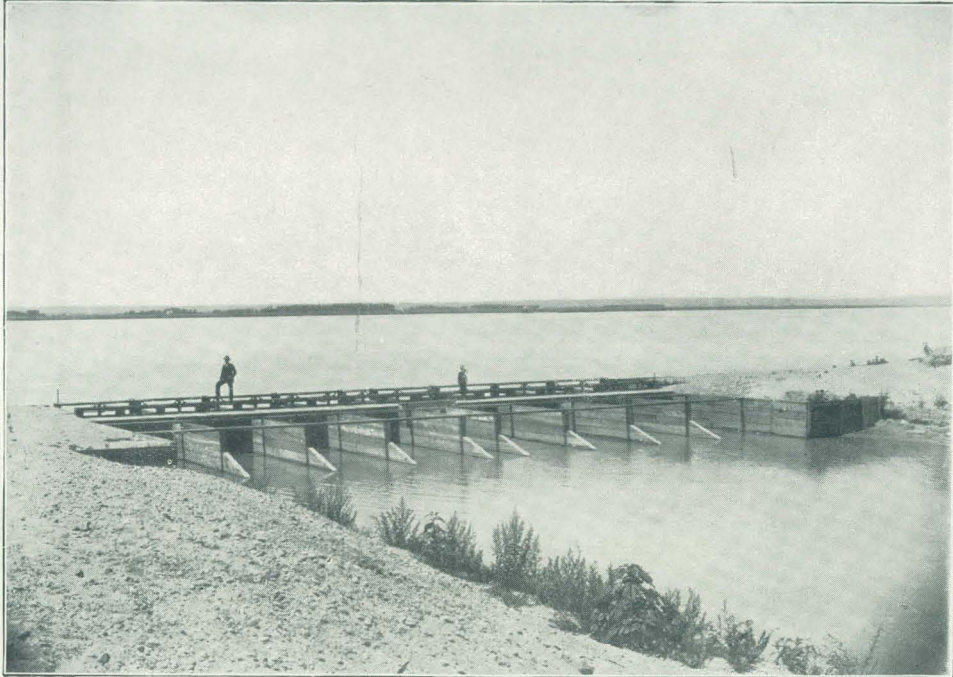
A. HEAD GATES OF CANAL OF FARMERS AND MERCHANTS IRRIGATION COMPANY ON PLATTE RIVER NEAR COZAD, NEBRASKA.
