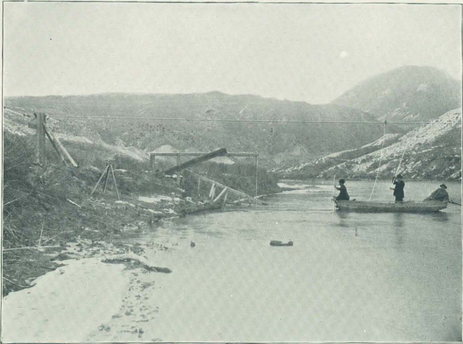
A. MEASURING BEAR RIVER AT COLLINSTON, UTAH.
