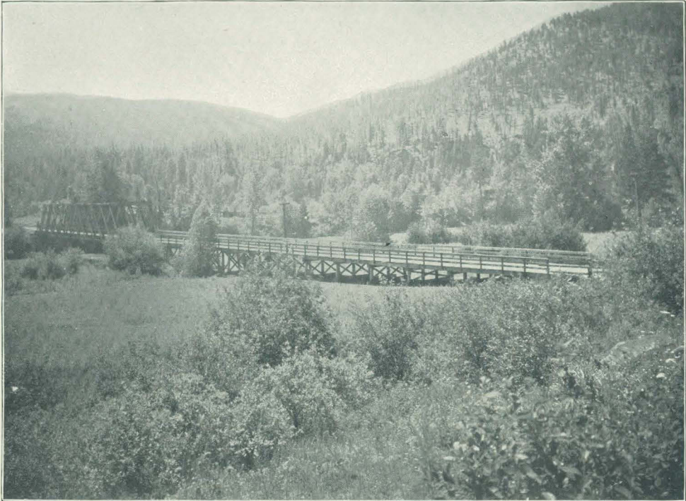
A. GAGING STATION ON BLACKFOOT RIVER, MONTANA.
