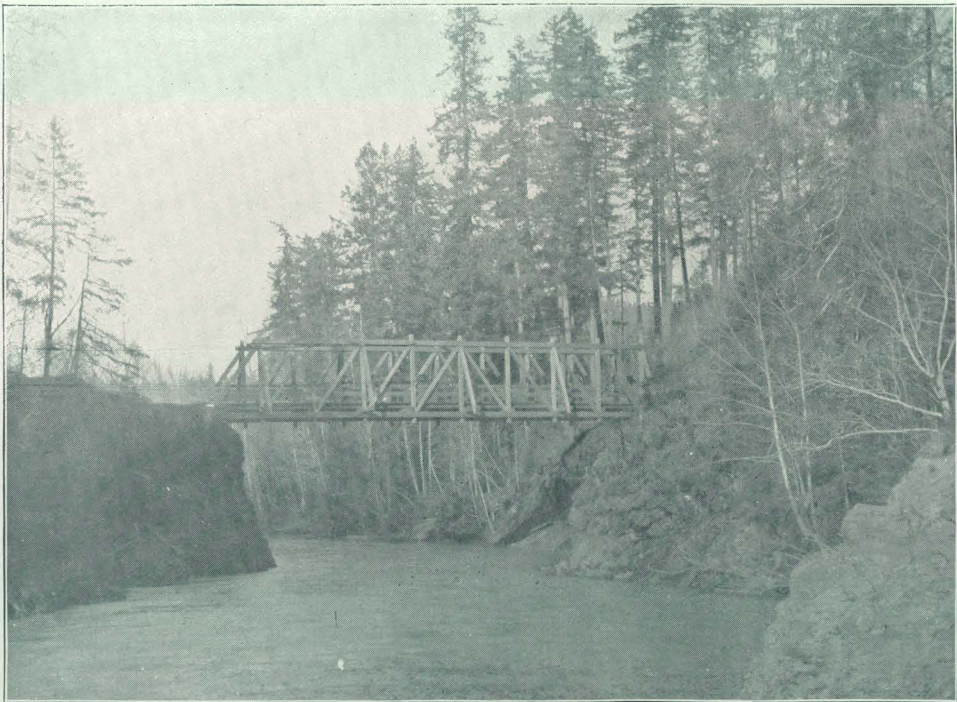
B. BRIDGE ACROSS ELWHA RIVER AT McDONALD, WASHINGTON.
