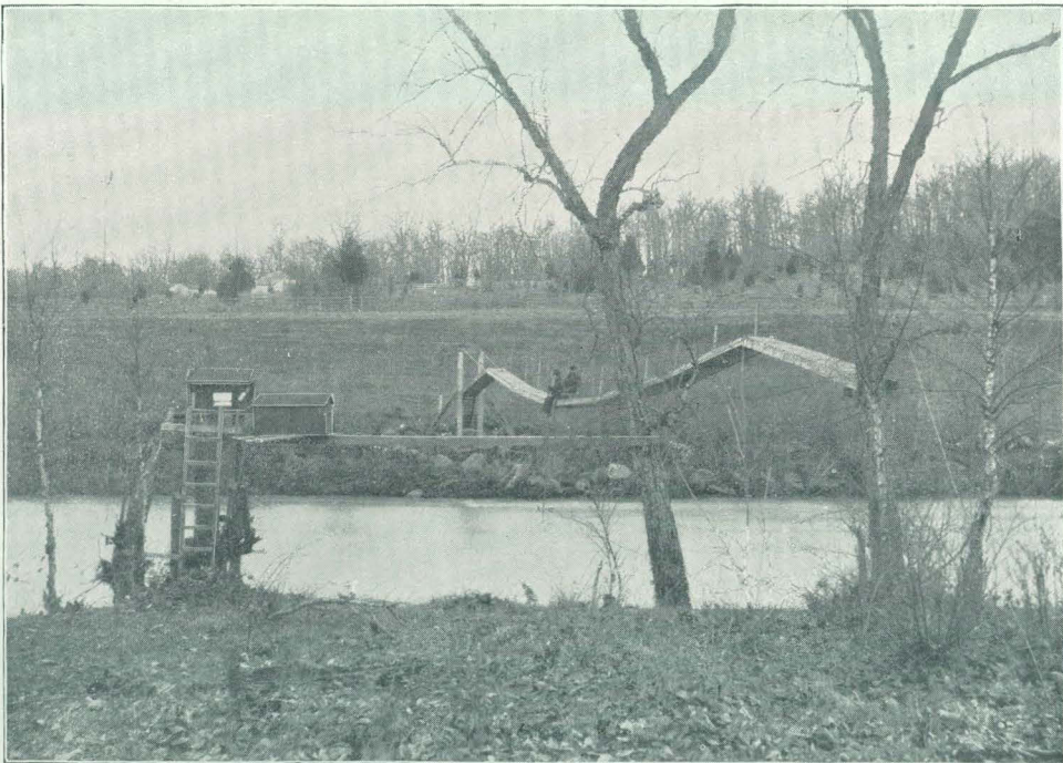
B. SUSPENSION BRIDGE AND NILOMETER ON PERKIOMEN CREEK AT FREDERICK, PENNSYLVANIA.
