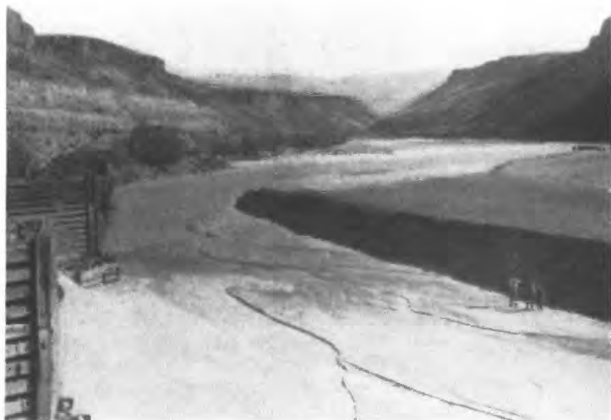
Deposition of sediment in irrigation canals and in parts of the Boise River channel, as above the Diversion Dam shown in the photograph, had increased maintenance costs in many canals since the mid-1920's. During an 18-month period in which Survey scientists measured the daily discharge and sediment loads in the drainage basin, they found that the sediment consisted largely of coarse material at stations above the active placer mines near Idaho City but entirely of fine material below the mines. They concluded that most of the coarse material passing the stations above Idaho City was deposited behind tailings from dredging operations in the placer mining area but that in earlier years when the spring runoff was greater a large amount of coarse material had been carried downstream, discharged into the Boise River, and deposited in the river channel or in the larger irrigation canals. Much of the fine material was carried through the canals and eventually deposited in diversion ditches or on farm land. (From S. K. Love and P. C. Benedict, 1948.)
