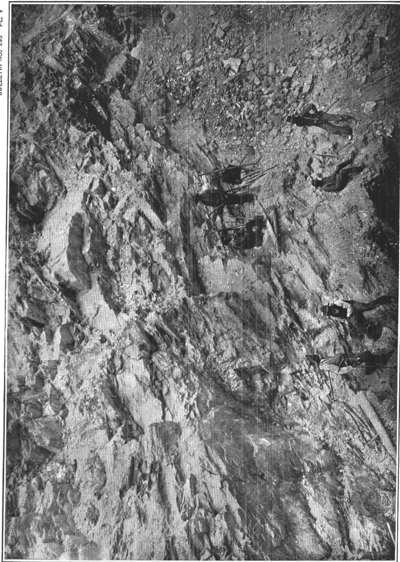
HAILE ORE BODY NEAR BOTTOM OF HAILE PIT. Showing foliation and dip. Looking northeast.
