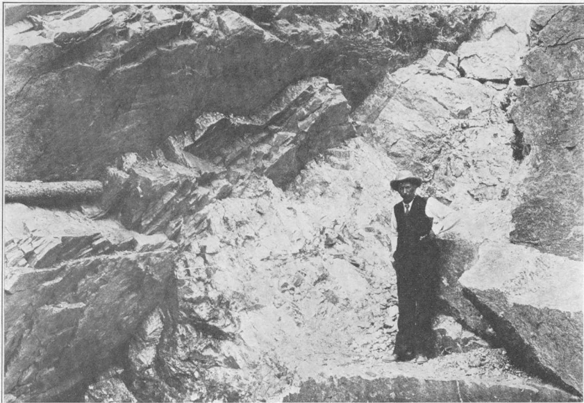
A. CONTACT OF PEGMATITE AND GNEISS IN NORTHEAST FACE OF OPEN CUT AT FIRESTONE MICA MINE, NEAR CUSTER, S. DAK.
